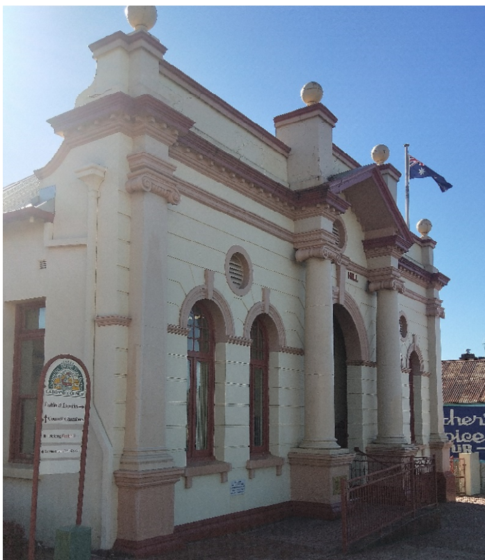
Cabonne Council's Molong Office
