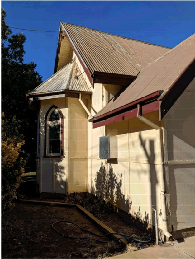
The front elevation noting the bay window and use of the Red and Cream. The joinery is to be restored. Elements of damaged fibro need to be replaced in compliance with WorkCover practice and the associated new cover battens.
