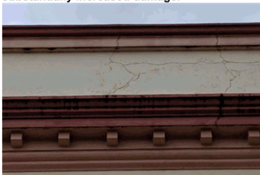
Image 3 The paint condition is considerably worse above the minor parapet. This may be due to the previous paint only reaching that lower level.
