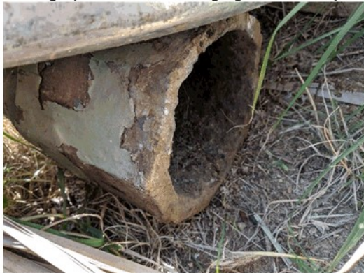
Photograph 6 Retained upper level post kept in the rear yard
