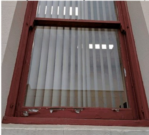
Image 8 The exposed timber is leading to rot and damaged to the primary timber sash and framing members.
