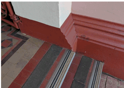
Figure 5 The entry where the coloured building base comes inside and hence continuity is required.
