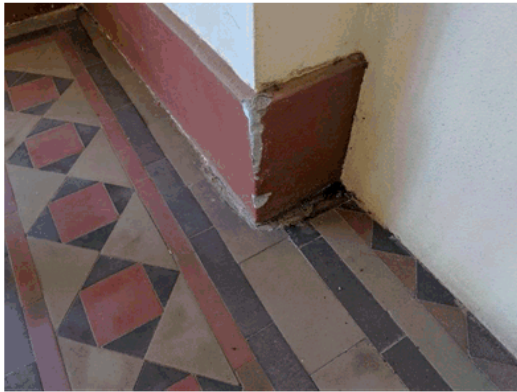
Figure 6 Another paint scrape area which reveals the cement render.
