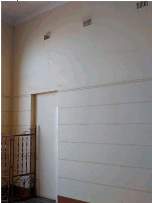
Figure 7 The walls to be painted to match the existing in the ashlar or rusticated faux stone are white in the flat area above, a half tint of the same colour can be used. this will lighten up the space and give transition to the ceiling white.
