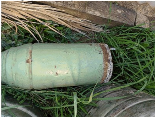
Photograph 5 Retained large ground floor post showing the base in the rear yard
