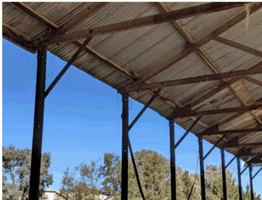
Photo 7 View to show the missing fascia and guttering on the East Elevation
