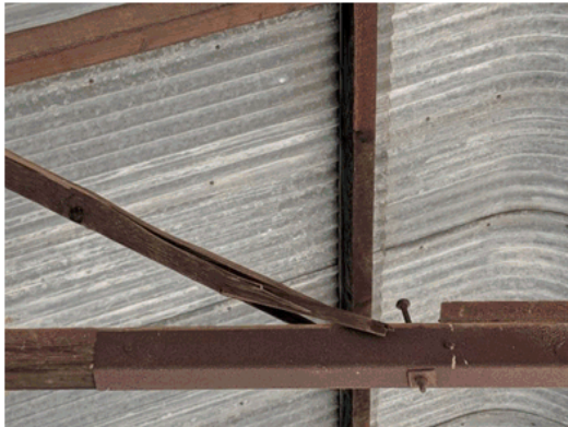
Photo 2 The damaged member causing the subsidence at Bay 16.
