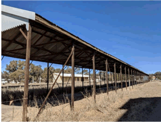
Photo 11 View along the West Elevation. Note the missing gutter and downpipes to 22 bays.
