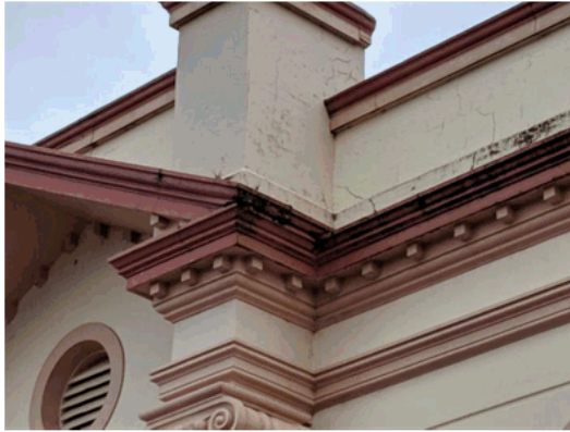
Image 2 Note the vegetation growth at the open joints in the cement features. The growth indicates gaps capable of water ingress and with frosts this will lead to substantially increased damage.
