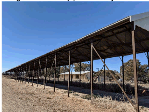
Photo 4 The West Elevation and the damaged gutter to 3 bays. There is no gutter to the other 29 bays
