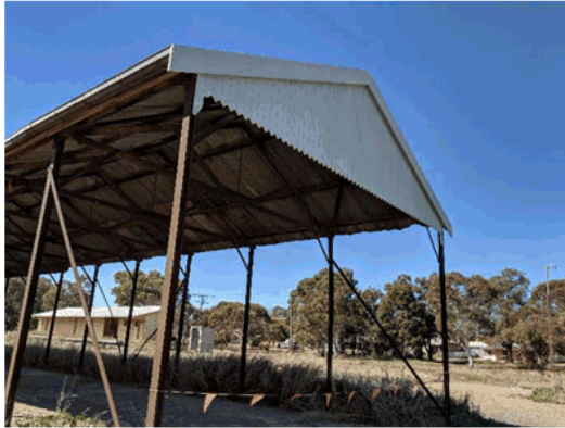
Photo 5 The reinstated timbering to the North end. Only the barge roll flashing to go plus paint.
