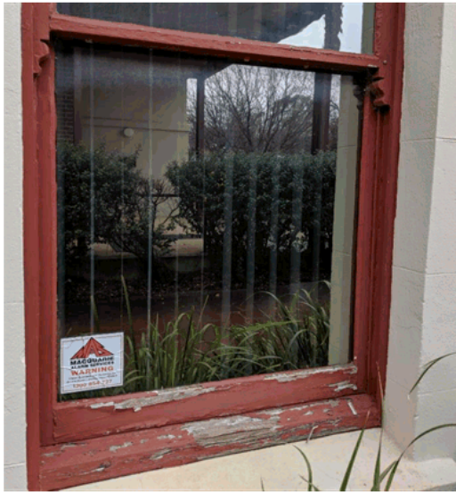
Image 9 The sills are the showing the greatest level of damage and decay. Note the ashlar treatment.
