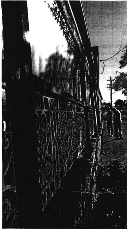
Photograph 3 View indicating the lean on the posts. The posts will need to be re-aligned to the vertical. This will determine the bearers beneath – new/existing/posts etc. The verandah should be independent of the stone work on new posts if possible to avoid future 'pull' away from the building by the subsidence action.
