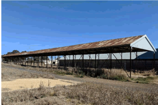
Photo 14 View of the East elevation and full 32 bays. Note the recently completed replacement of the gable end timbering to the North Elevation. Only the flashing and final painting is to be completed. The works are a great improvement and will increase the structural stability of the structure.
