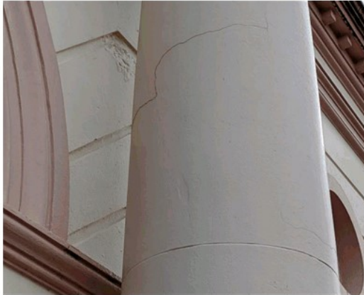
Image 7 Note the salt damage/bubbling in the ashlar details around the arches. Successive heavy paint coatings conceal the ashlar details. These reflect the decorative stone layout – ashlar. They can be re-scored prior to painting.
