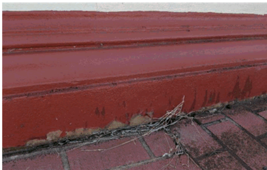
Figure 4 Also a good example of an earlier if not original paint colour is this area where the paint has been scraped off.
