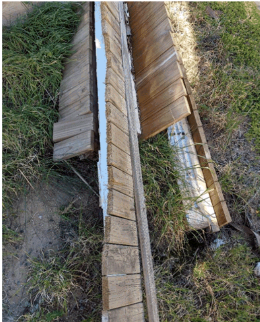
Photograph 3 Remnants from the first floor. Noted that this material was decking and was treated pine. Traditional verandah floors are cypress tongue and grooved flooring which is not decking. The traditional flooring would be specified in the verandah reinstatement.
