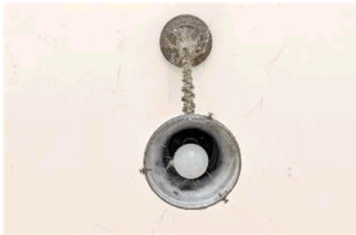
Figure 9 The fitting indicates a standard incandescent lamp which is nominally 5cm in diameter and therefore the throat on the brass gallery is nominally 14-15cm wide which would accept a glass with a 5" neck.
