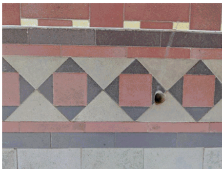
Figure 2 A direct view of the tessellated floor tiles. The dark brown rectangular border tile is a good marker for selecting an appropriate colour for the cement rendered skirting and building base.
