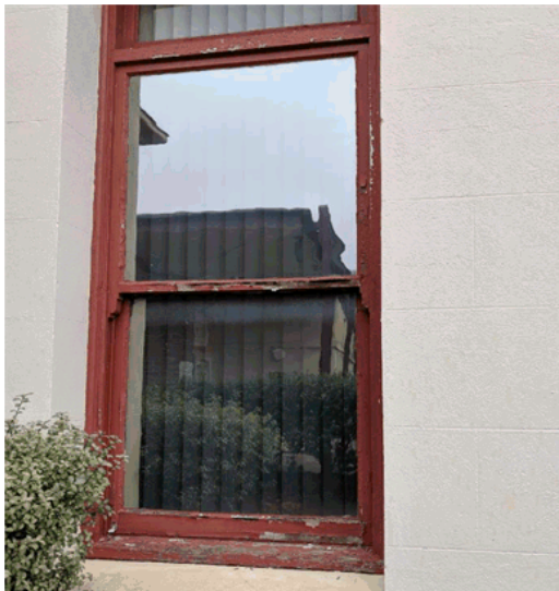
Image 10 The exposed timber is leading to rot and damage to the primary timber sash and framing members.
