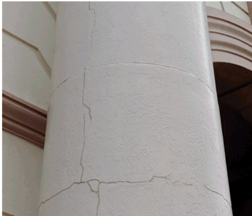
Image 6 The surface cracking in the two large columns on the front elevation is a cause for concern. Costs will increase exponentially should this damage not be restored to prevent water ingress.
