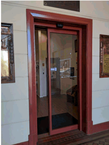
Figure 1 View of the building entry. The door is to be replaced with a frameless entry door. A colour is required for the architrave which will remain, the foot blocks and the skirting.
