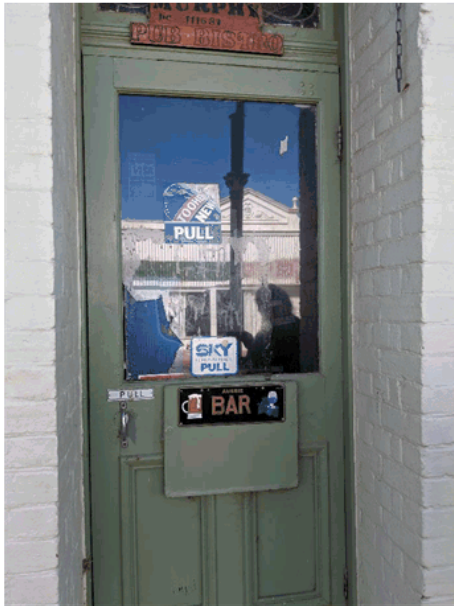
Photograph 7 The damaged glass pane in the side door which was damaged by vandals
