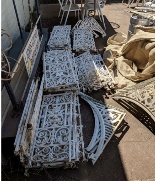
Photograph 2 Retained cast iron brackets in the rear yard. They will require thorough stripping before preparation, painting and reinstallation. The new installation will also need to comply with current regulations which will require a new verandah floor mounting detail to ensure that the handrail meets the height requirements established by the current BCA.
