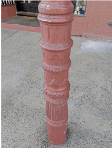
Photograph 8 Existing retained cast iron post in the footpath. Note the different base or encapsulation.
