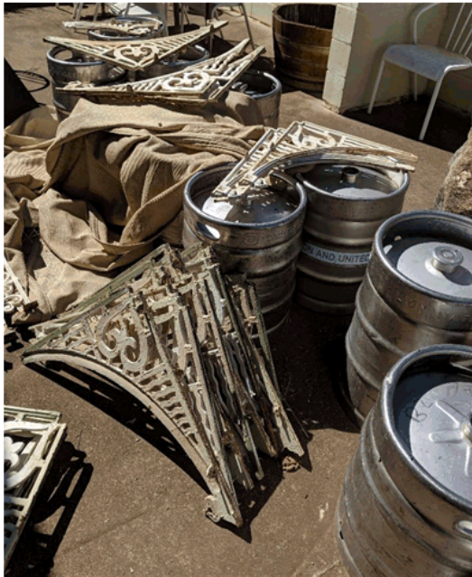
Photograph 1 Original retained brackets in the rear yard. They are generally sound and in good condition subject to cleaning.
