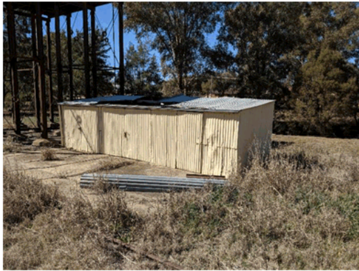
Photo 15 The Fettle's shed, noting the missing roof sheets. These are on the ground in the vicinity and may have been blown off in a storm event.
