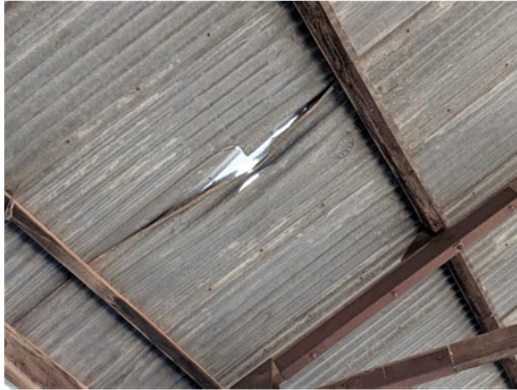
Photo 8 Damaged roof sheeting. Generally the most damage is to the East side and tallies up to 5 areas and 45m 2 of sheeting. One area is curved at the ridge which could be rolled and restored. All the sheeting requires a preparation and coating of Fisholene. Access is an issue requiring a large boom lift.
