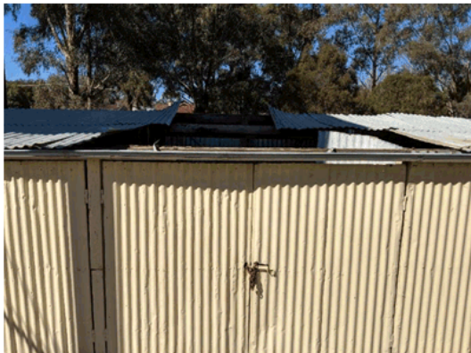
Photo 16 Close view illustrating the size of the open roof and exposed timbers.
