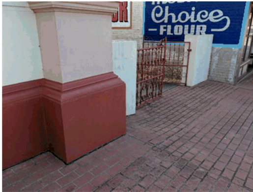
Figure 3 The building base and side entry
