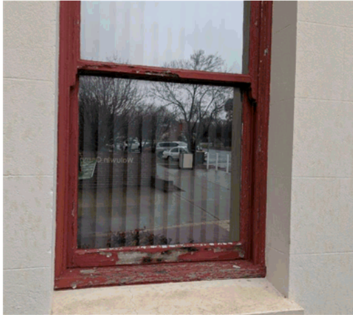
Image 11 The exposed timber is leading to rot and damage, expressed above in the fungal black staining to the primary timber sash and framing members.
