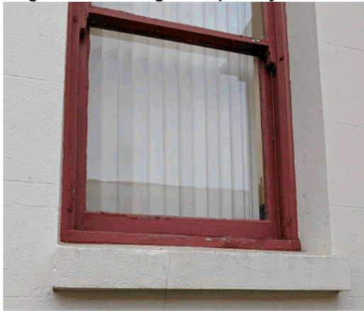
Image 12 The exposed timber is leading to rot and damaged to the primary timber sash and framing members. Note the cracking line from the wall through the window sill.
