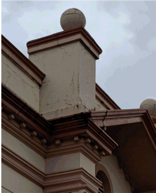
Image 5 Note the open joints in the pediment and the general surface cracking in the render.
