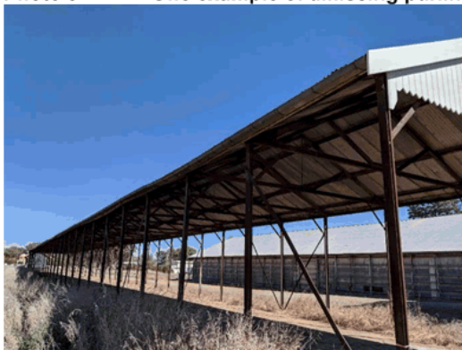
Photo 10 The East Elevation with damaged gutter. Restoration is possible but may not be viable.
