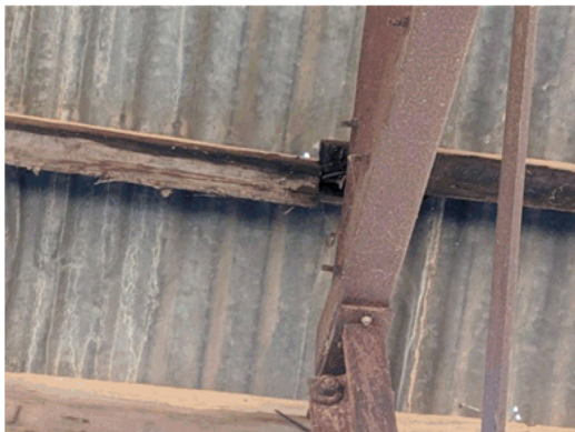
Photo 9 One example of a missing purlin.
