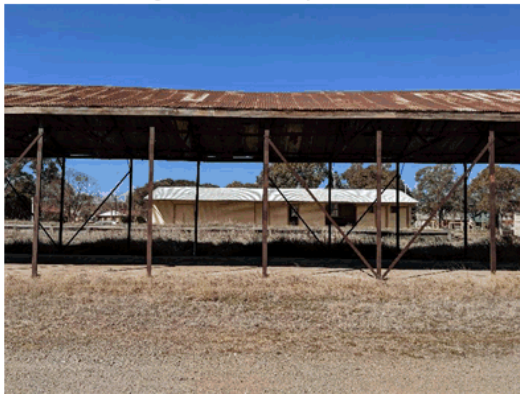
Photo 1 The central bay No.16 of 32 bays where the timber roof truss has a broken member and hence the roof subsidence evident in the photo.
