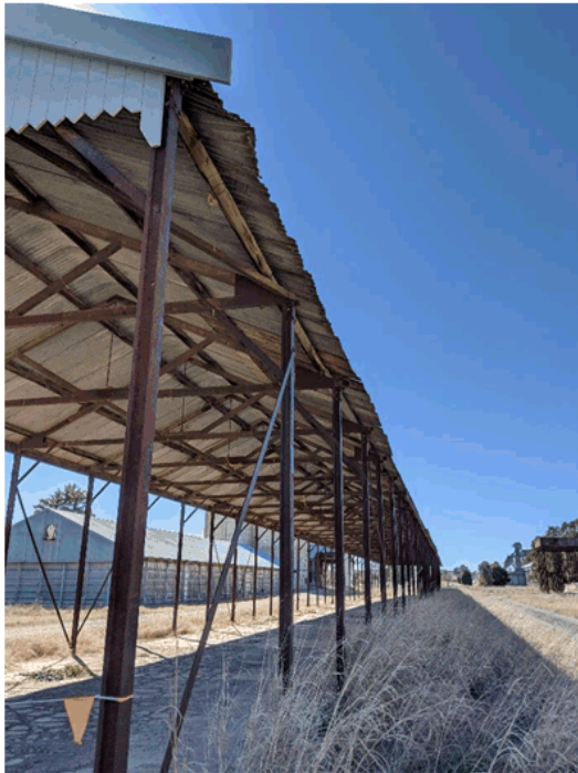
Photo 3 View along The East Elevation with missing timber fascia and galvanised steel gutter and downpipes to 16 bays
