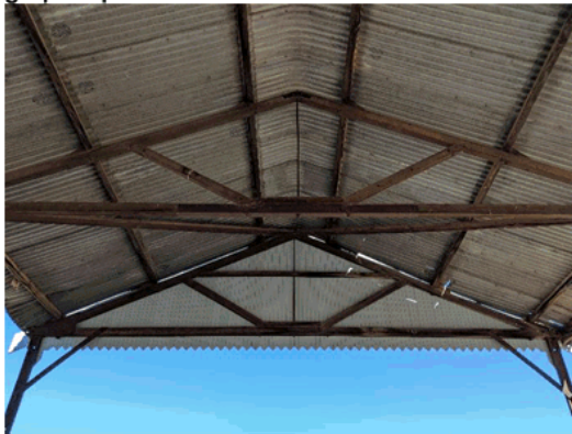
Photo 6 Note the gaps and damaged roof sheeting where the flashing will be reinstated.
