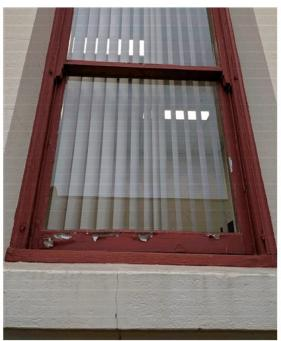
Image 8 The exposed timber is leading to rot and damaged to the primary timber sash and framing members.
