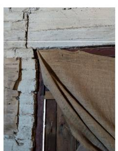
Figure 3 A Detail view of the movement cracks in the lintel. The lintel appears to be a poured in place concrete beam and will be heavy at this scale. In addition the lintel appears to have insufficient bearing on both sides of the opening.
