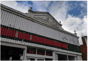
Photo 11 The cement rendered pediments are highly significant remnants and it is hoped that similar elements remain beneath the cladding
