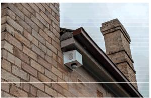
Photograph 10 Review the missing gable infill and repair. Re-point the top set of bricks on the chimneys.
