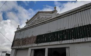
Photo 10 The 'super-six' asbestos cladding needs to be removed by a licensed asbestos contractor and the premises then tested.
