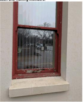
Image 11 The exposed timber is leading to rot and damage, expressed above in the fungal black staining to the primary timber sash and framing members.
