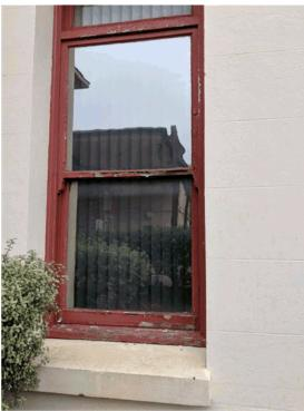
Image 10 The exposed timber is leading to rot and damage to the primary timber sash and framing members.
