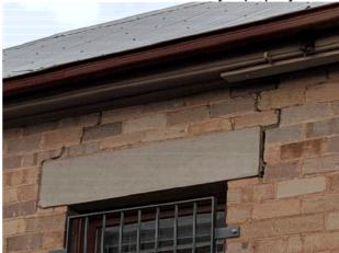
Photograph 7 Previous cement re-pointing should be replaced with lime mortar to avoid brick damage. Engineer to inspect the lintels as they appear to have moved away and out from the wall face.
