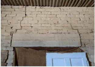
Figure 2 Interior view of the original skin of brickwork and lintel. The two cracks illustrate a number of possible scenarios:
