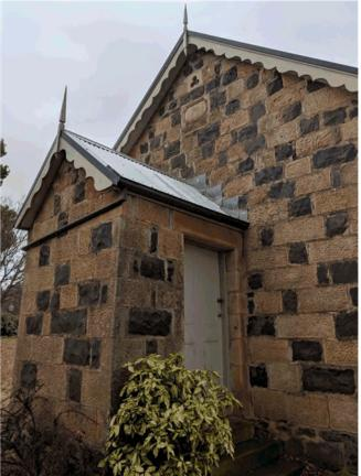
Picture 5 The key former frontage to the Church, noting the plants and vegetation which should be cleared from the building stonework to reduce the risk from rising salt damp.
