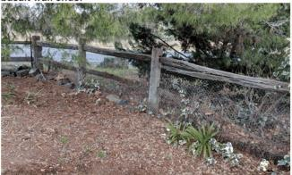
Picture 2 The general run of post and slotted timber fence. This fence is possibly rare and significant.
