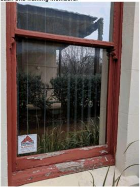
Image 9 The sills are the showing the greatest level of damage and decay. Note the ashlar treatment.
