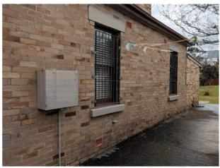
Photograph 2 Side elevation. The bars on the windows detract from the heritage significance. 'Crimsafe' or 'Securimesh' would be a better deterrent and enhance the character as they read as a screen. Otherwise the condition appears fine.
