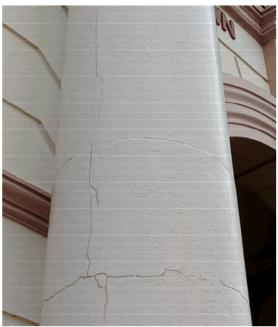
Image 6 The surface cracking in the two large columns on the front elevation is a cause for concern. Costs will increase exponentially should this damage not be restored to prevent water ingress.
