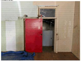
Photo 6 A simple but bold industrial feature worthy of retention even if for fire reasons it needs to be relocated so that a Code compliant door needs to be installed.
