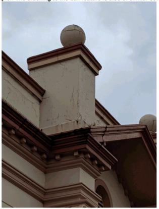
Image 5 Note the open joints in the pediment and the general surface cracking in the render.
