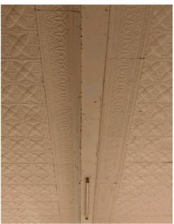
Photo 7 The pressed metal ceilings are generally sound in the front portion. A review of the ceiling space and weatherproof status of the roofing will reveal the issues. All the lighting needs to be replaced to reduce energy consumption and for installing appropriate heritage quality fittings.
