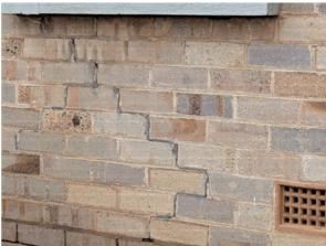
Photograph 8 Previous cement re-pointing should be replaced with lime mortar to avoid brick damage.
