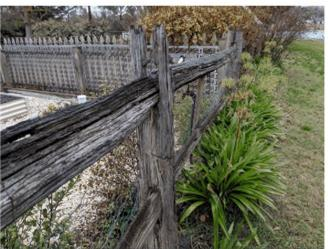
Picture 7 Recommend restoration of the fencing and replacement of timbers not capable of being restored and reused. Do not modernise this structure given its rarity and retain the structure for as long as it can be kept standing. For example the split rails can be bound with galvanised fencing wire to prevent further splitting.
