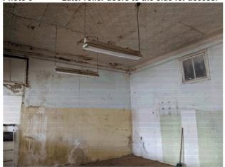
Photo 4 The rear room with the rusty ceiling, apparently due to the storage of wet hay/lucerne products. The current concept is to use this space for new toilets in part due to the advanced decay. The first step is to investigate the extent of the decay as part of a general condition audit for the whole site/buildings. This document can then be used to review alternate concepts for meeting the brief.
