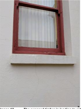
Image 12 The exposed timber is leading to rot and damaged to the primary timber sash and framing members. Note the cracking line from the wall through the window sill.
