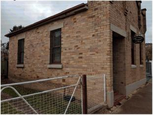
Photograph 6 Evidence of rising damp is the loss of the lower bed joints in the brickwork. Pointing using a lime based mortar is required.
