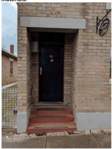
Photograph 5 The entrance will not comply with the AS or DDA Act for access. In view of the building size and conservation area setting, an alternate solution will be possible to another entry point. A report justifying this approach with the solution illustrated will be required.
