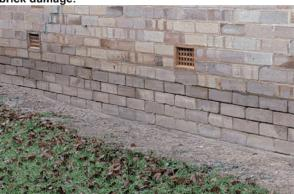
Photograph 9 Note the loss of the mortar from the bed joints due to rising salt damp. Refer to the advice on rising salt damp and re-pointing in lime based mortar and the edge pathway
