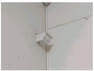
Photo 9 Timber corbel brackets which were regularly spaced at a specific level in the Department Store rooms. Visit the Up to Date store in Coolamon, as an intact example of the building type. The brackets may have been part of a shelving system, a cash carrying system or a lighting system. Restoration of the existing and identifying them on the walls even where removed in order that they can be interpreted, is recommended.
