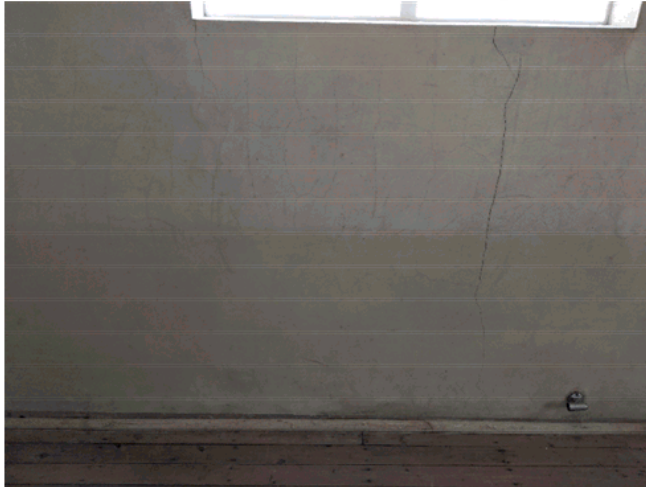
Internal wall illustrating the watermark from a previous flood event
