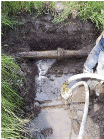
Trunk water main repair
