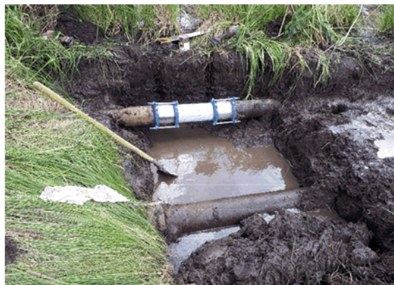
Trunk water main repair
