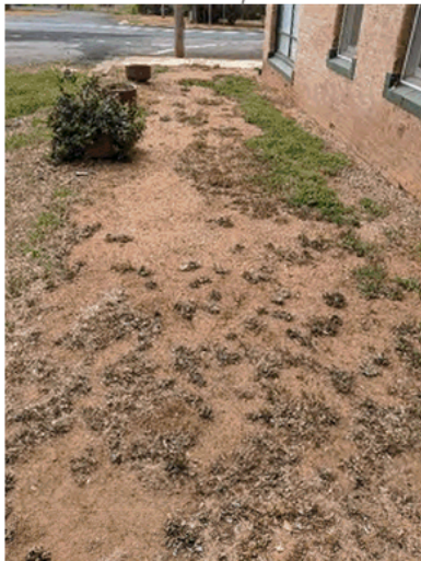
Side area requiring a consolidation and grading to fall
