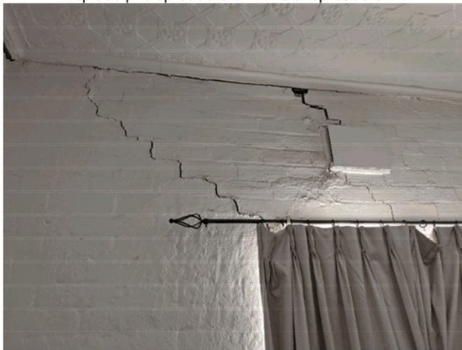
Internal cracking which requires reconstruction or stitching
