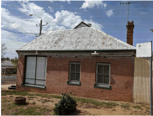
General view of the North Elevation
