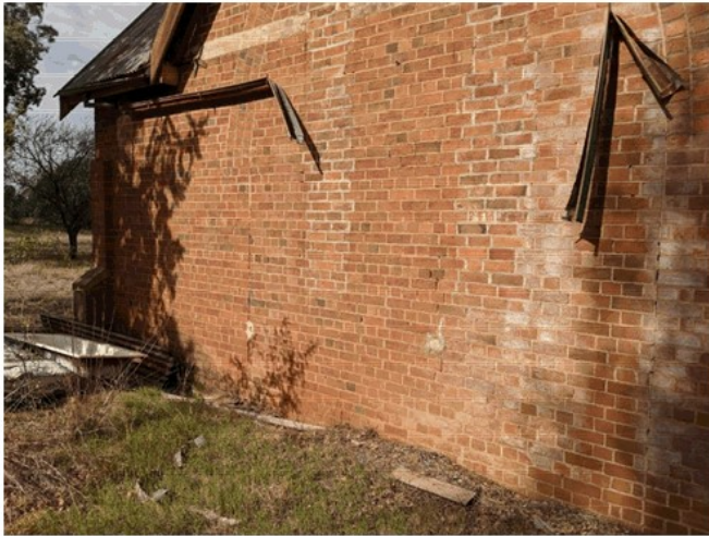
West elevation of the west wing noting the infilled two lancet windows These can be reinstated
