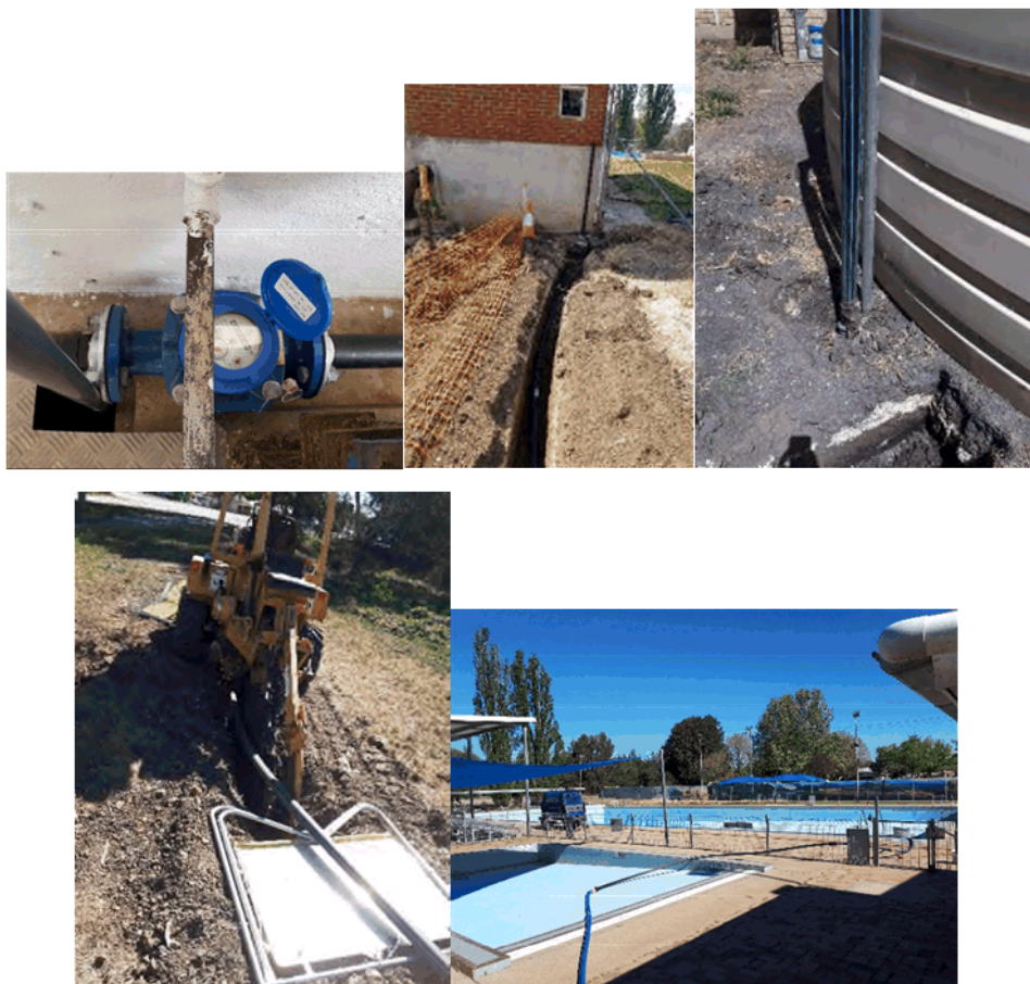
Infrastructure – groundwater utilization at Molong, Cumnock and Manildra pools.
