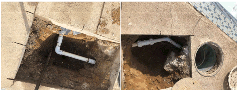
Eugowra pool painting, Eugowra re-tiling, toddlers & main pool, Eugowra major water leak repair.
