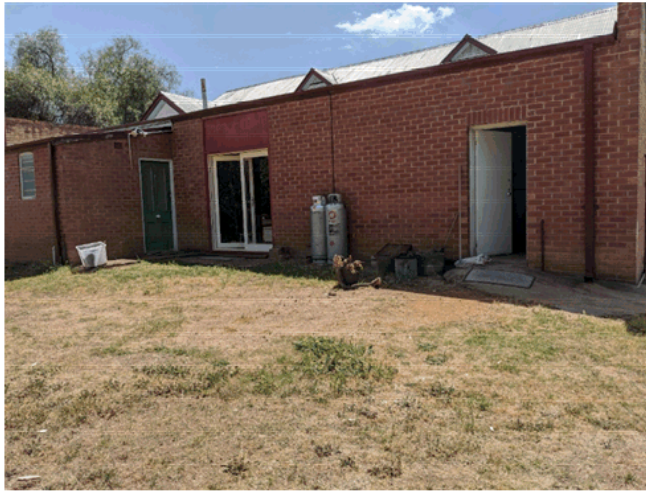
Rear elevation: Note location of gas bottles within the flood prone area and three sets of doors which could be banded for protection.
