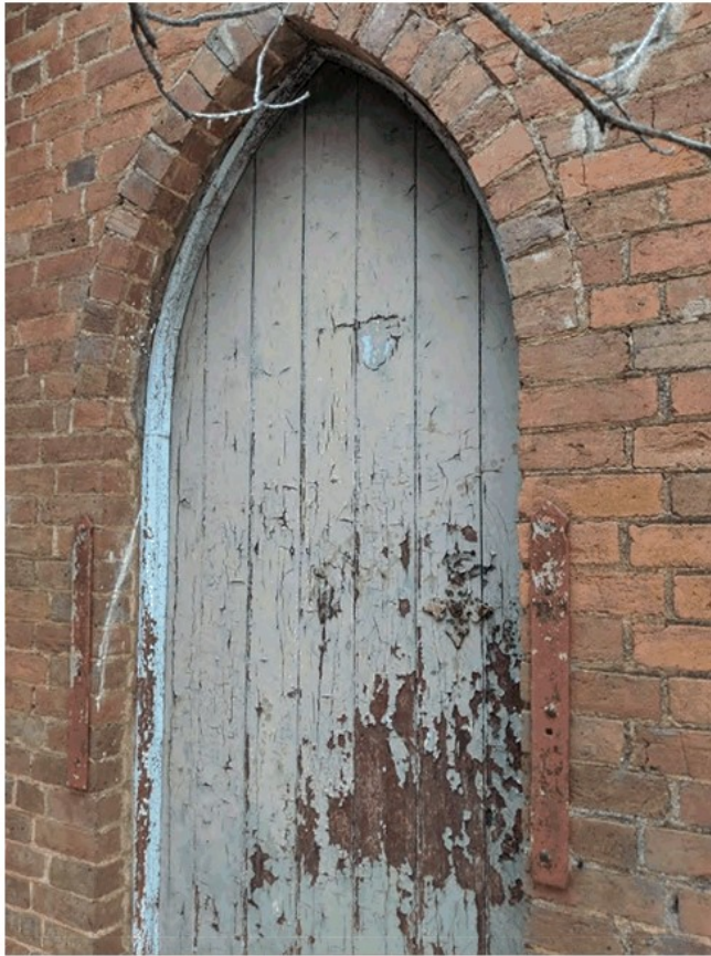
The original and remaining Church entry door with gothic details
