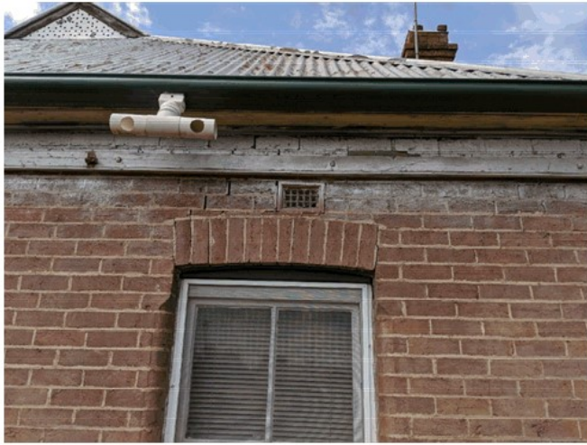
Damaged brickwork – review repair options and paint removal Replace pvc spreaders with metal spreaders
