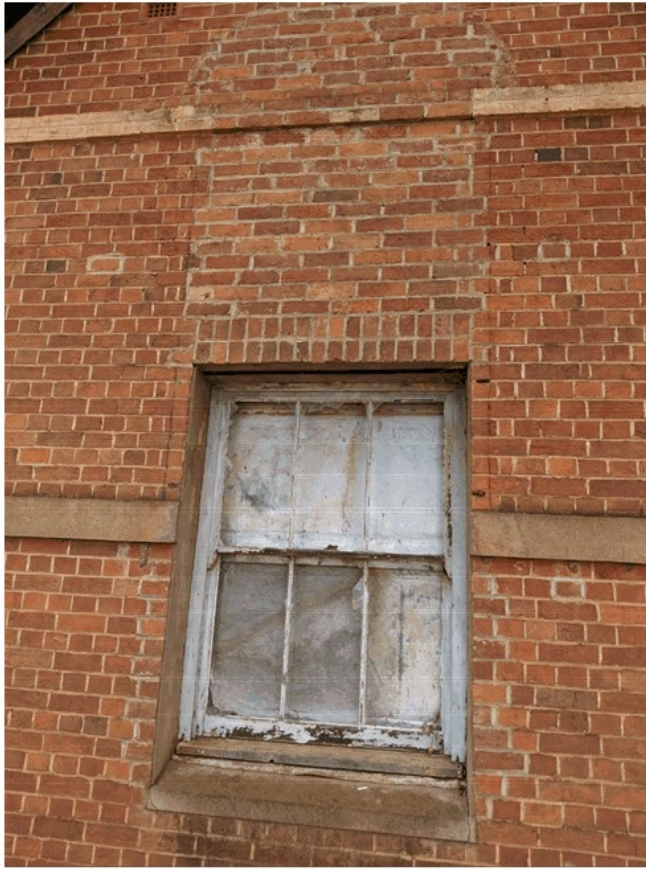
Infilled window in the north face of the west wing. This area recommended for adaptation into a door and link through to the extension
