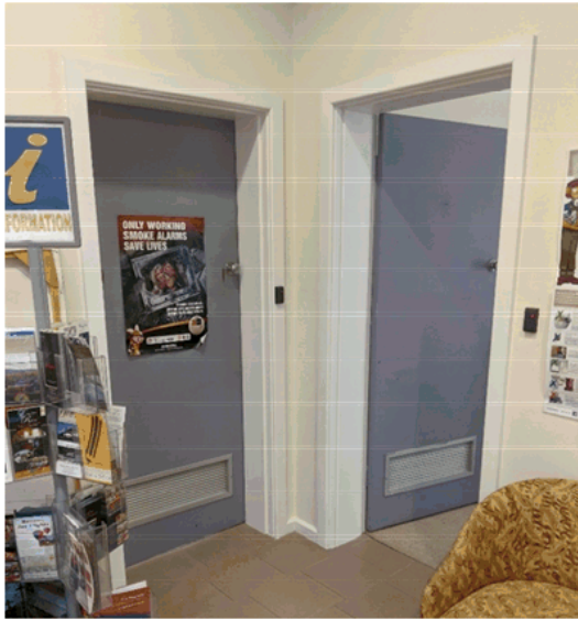
View of the doors, skirtings and architraves
