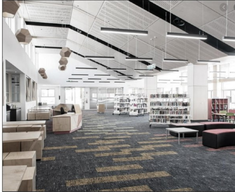
FEATURE ACOUSTIC CEILINGS ON RAKED CEILING WITH GAPS FOR CEILING SERVICES PLANK CARPET TILES
