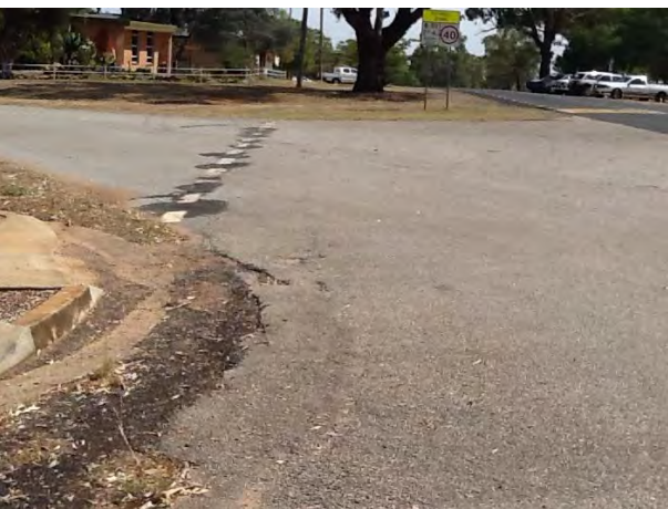
Corner of Bathurst Street and Forbes Street
