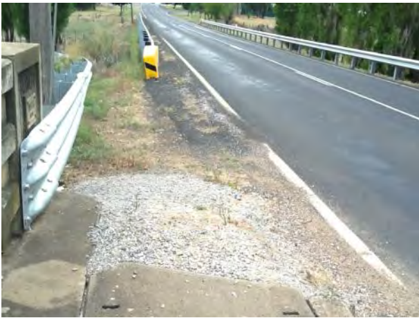
Pedestrian access to Boree Creek bridge (eastern approach)
