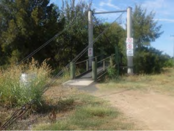
Southern approach to swinging footbridge
