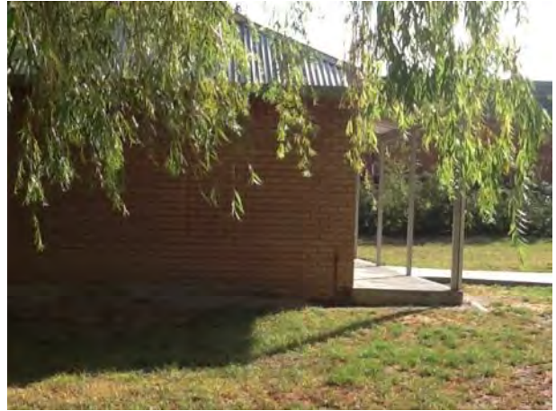
No footpath linking the footbridge and the toilet block
