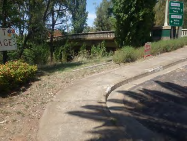
Accessing the bridge on both sides of the western approach involves traveling towards the road traffic before a sharp and narrow turn onto the bridge's footpath
