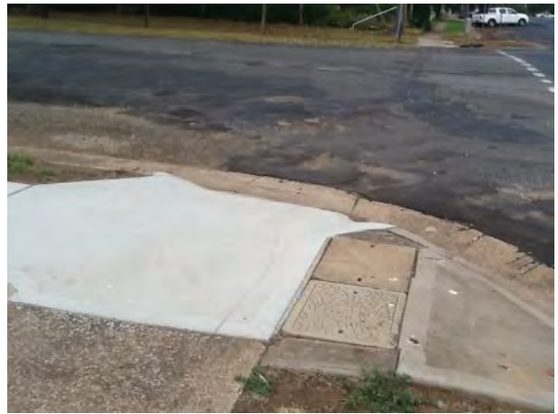
Smith Street near Main Street in the roadway at crossing point
