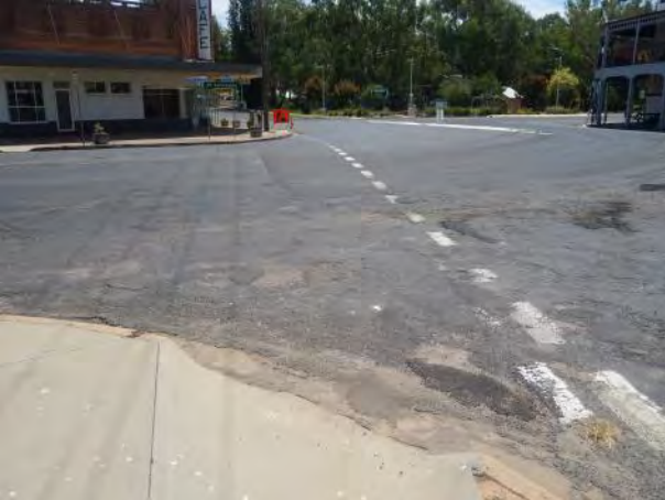
Corner of Pye Street and Nanima Street
