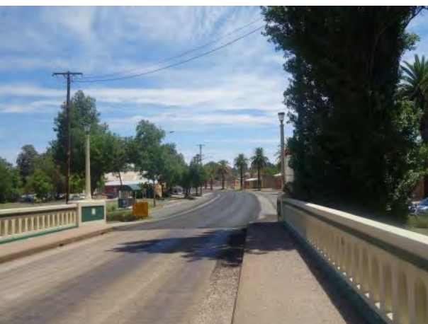
Footpath on bridge adjacent to vehicle traffic
