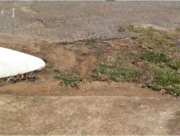
King Street and Forbes Street
