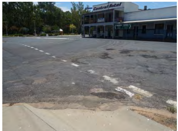
In roadway at crossing point, Nanima Street and Pye Street
