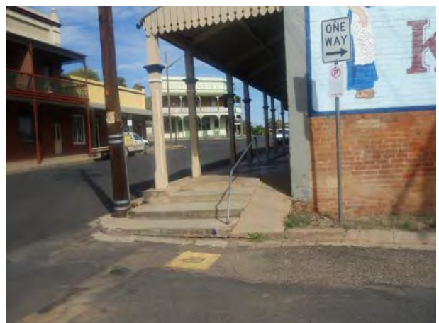
Kerb on Gaskill Street near laneway to swinging footbridge
