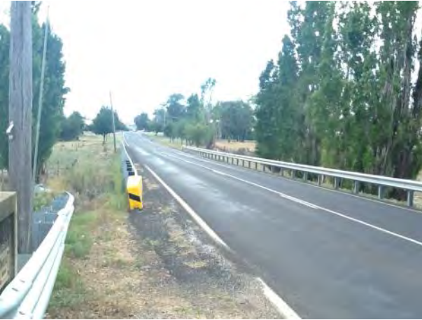
Boree creek bridge (western approach)
