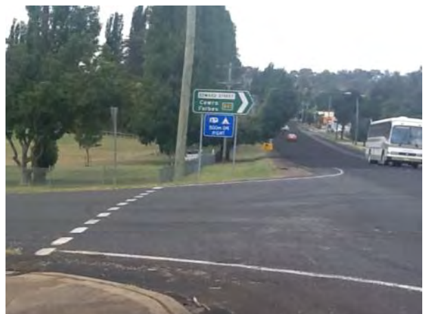
Hill Street adjacent to recreation ground
