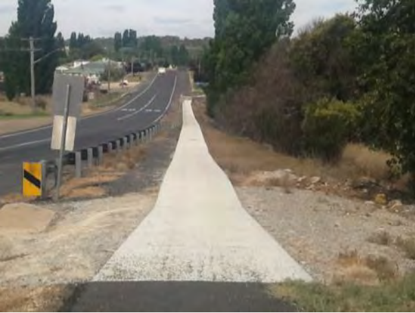
Hill Street near Kite Street (link needed between kerb ramp and Hill Street path)
