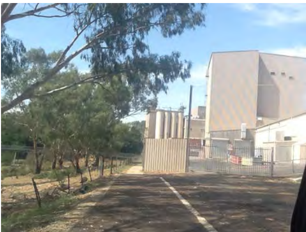
Footpath conflicts with mill driveway at eastern end of Loftus Street
