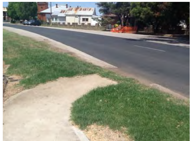
Southern side of Obley Street bridge (footpath over bridge only on eastern side)
