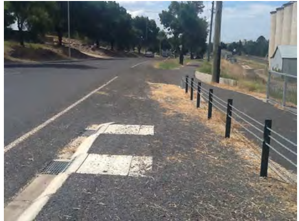
Watson Street near Wellington Street – no separation from vehicles
