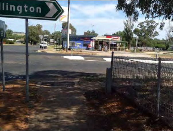
Forbes Street and Obley Street
