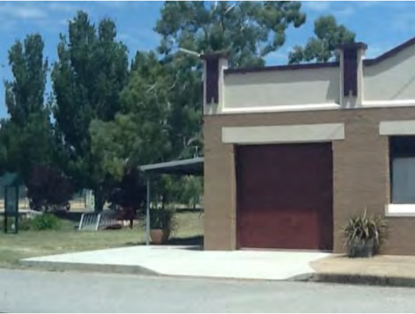
Between Obley Street and the footbridge
