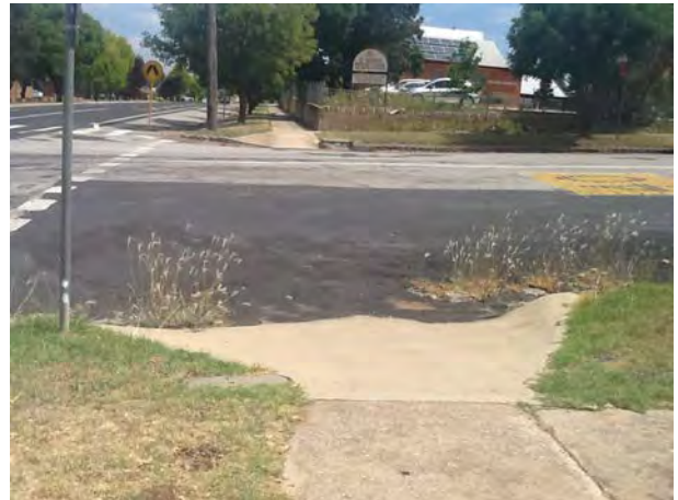
Edward Street and Riddell Street north west corner
