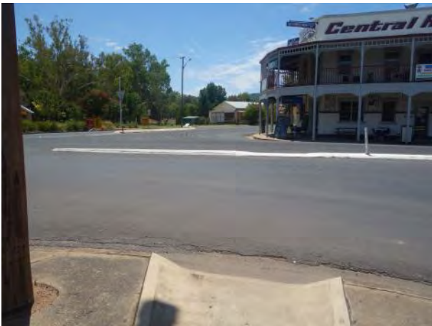
Narrow pedestrian refuge at the intersection of Nanima Street and Pye Street
