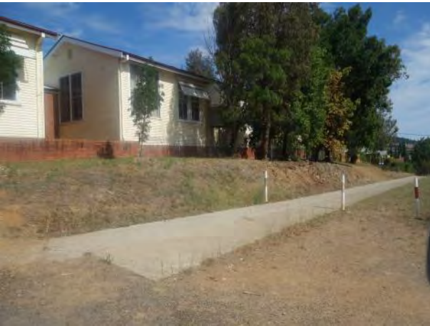
Tigla Street footpath becomes loose gravel near entrance to public school
