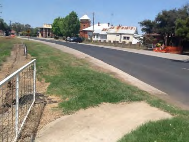
Narrow footpath on eastern side of Obley Street south of bridge
