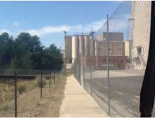
Access to footbridge from Loftus Street
