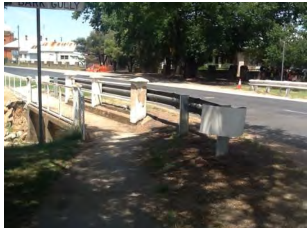
Access to the footbridge
