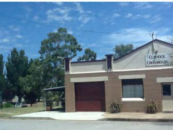
Obley Street where the shared path ends at the park
