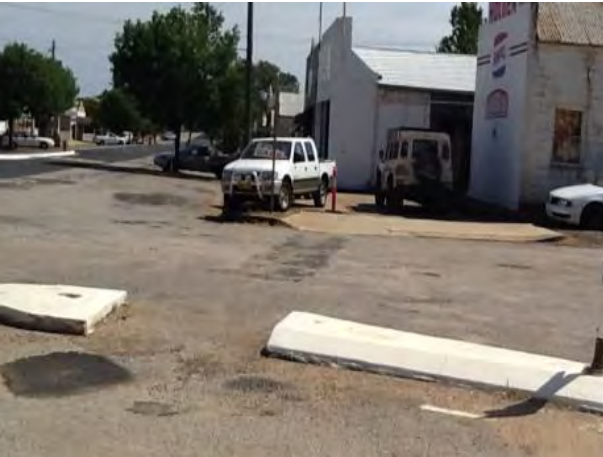
Narrow pedestrian refuge on King Street
