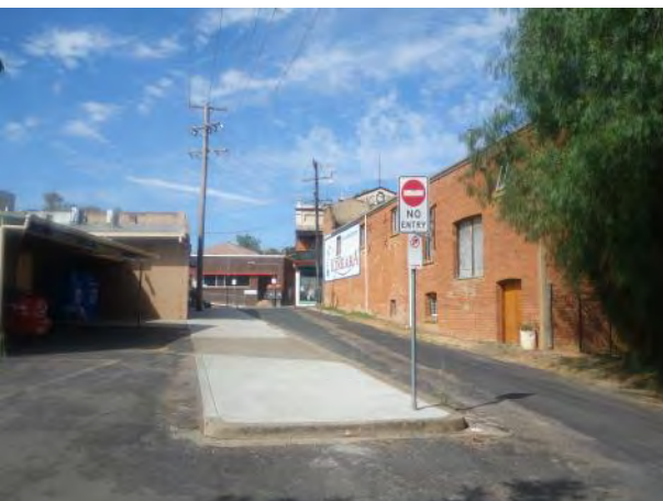
Kerb in laneway to/from swinging footbridge from Gaskill Street
