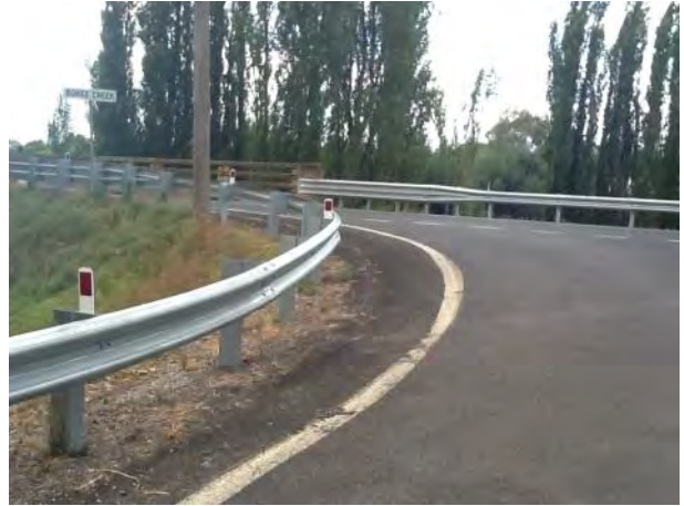
On approach to Boree Creek bridge from Merga Street
