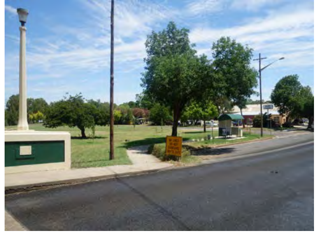
Lack of safety barrier on approach to Broad Street bridge (western approach, southern side)
