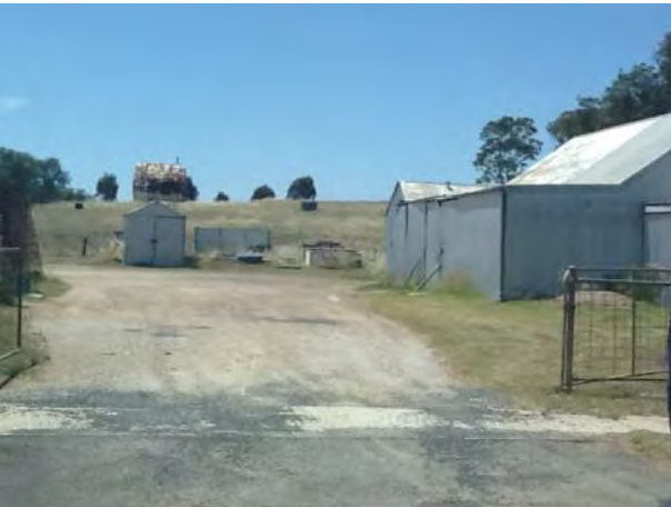
Obley Street driveway
