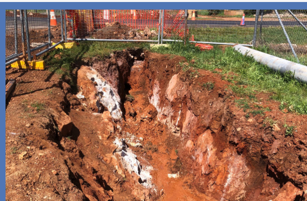
Molong Bore Project in progress
