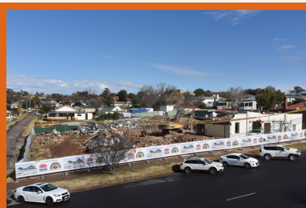
Demolition commenced on Molong Community Hall
