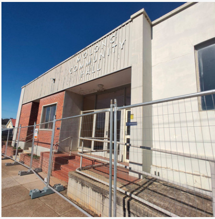
Demolitions begin at the Molong Community Hall
