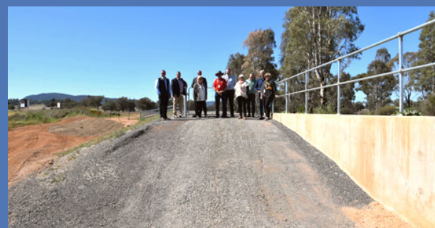
The completed Puzzle Flat Creek flood levee
