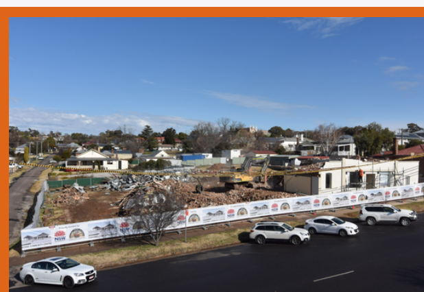
Demolition commenced on Molong Community Hall
