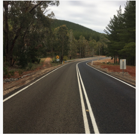
Four Mile Creek road upgrade
