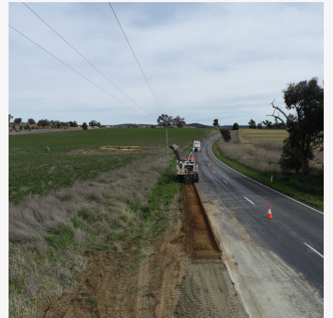
Henry Parkes Way road upgrade
