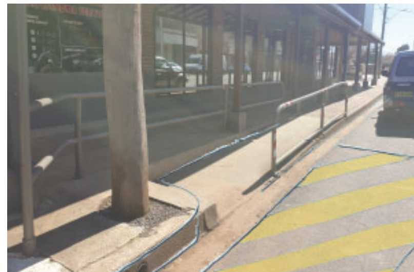
Remove sharp corners from ramp ends in Gaskill Street and paint no parking zones on the street surface, to alert drivers not to block exits.
