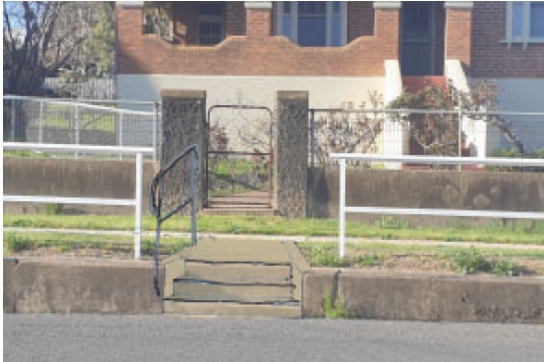
Cut compliant steps into existing step locations off the eastern end of Gaskill Street, and provide compliant handrail.
