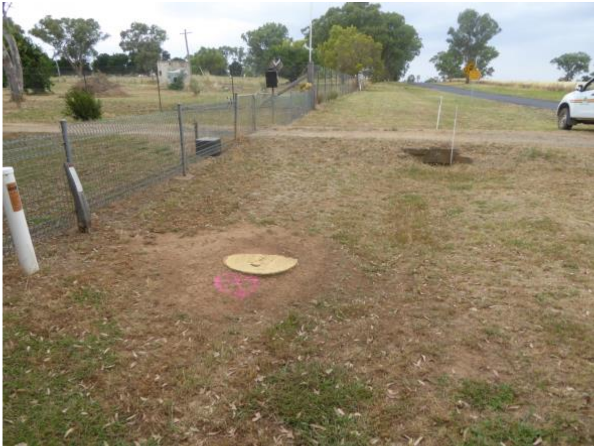
PLATE 15: Line 8A – View of the alignment, looking south from the vicinity of the peg at Ch. 0.0m (hydrant).
