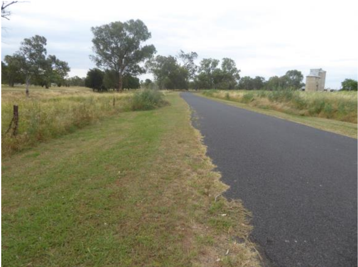
PLATE 10: Line 5A – View of the alignment, looking north-west, from the vicinity of the intersection of Railway Parade and Renshaw McGirr Way.
