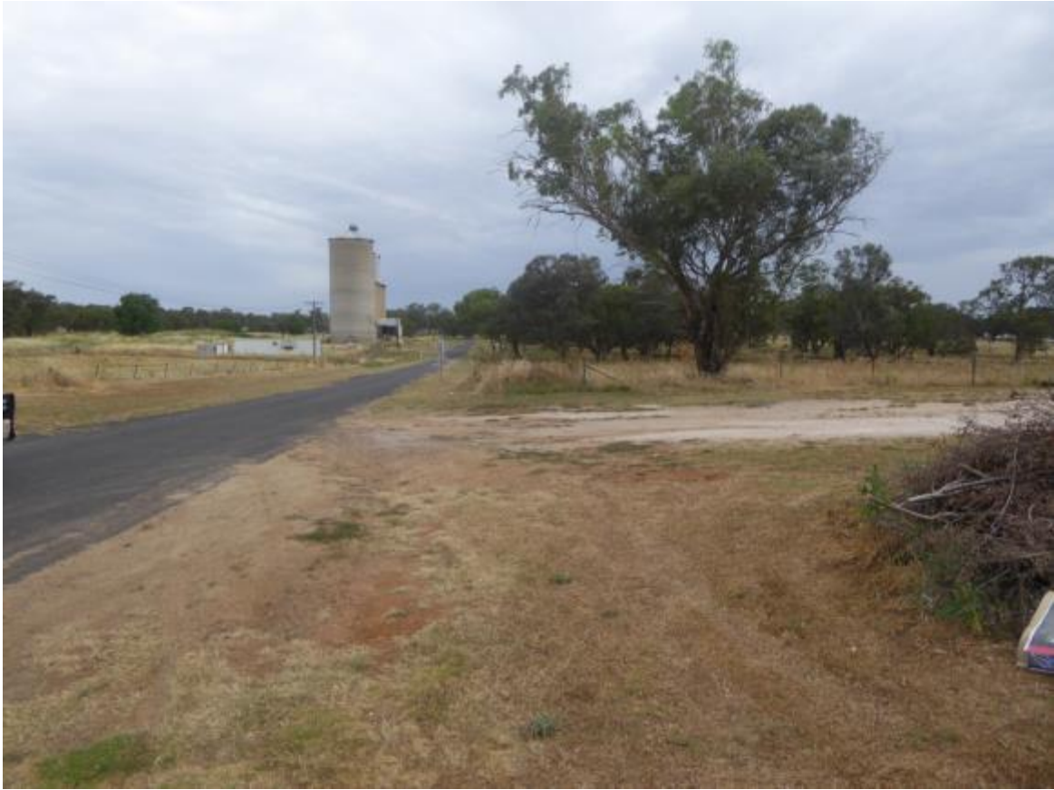
PLATE 11: Line 5A – View of the alignment, looking south from the vicinity of borehole BHY18.
