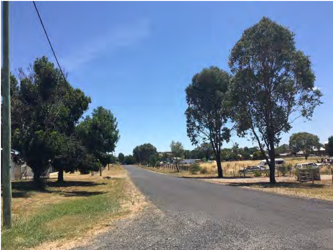
Plate 12: Section 2 (Cumnock) facing north
