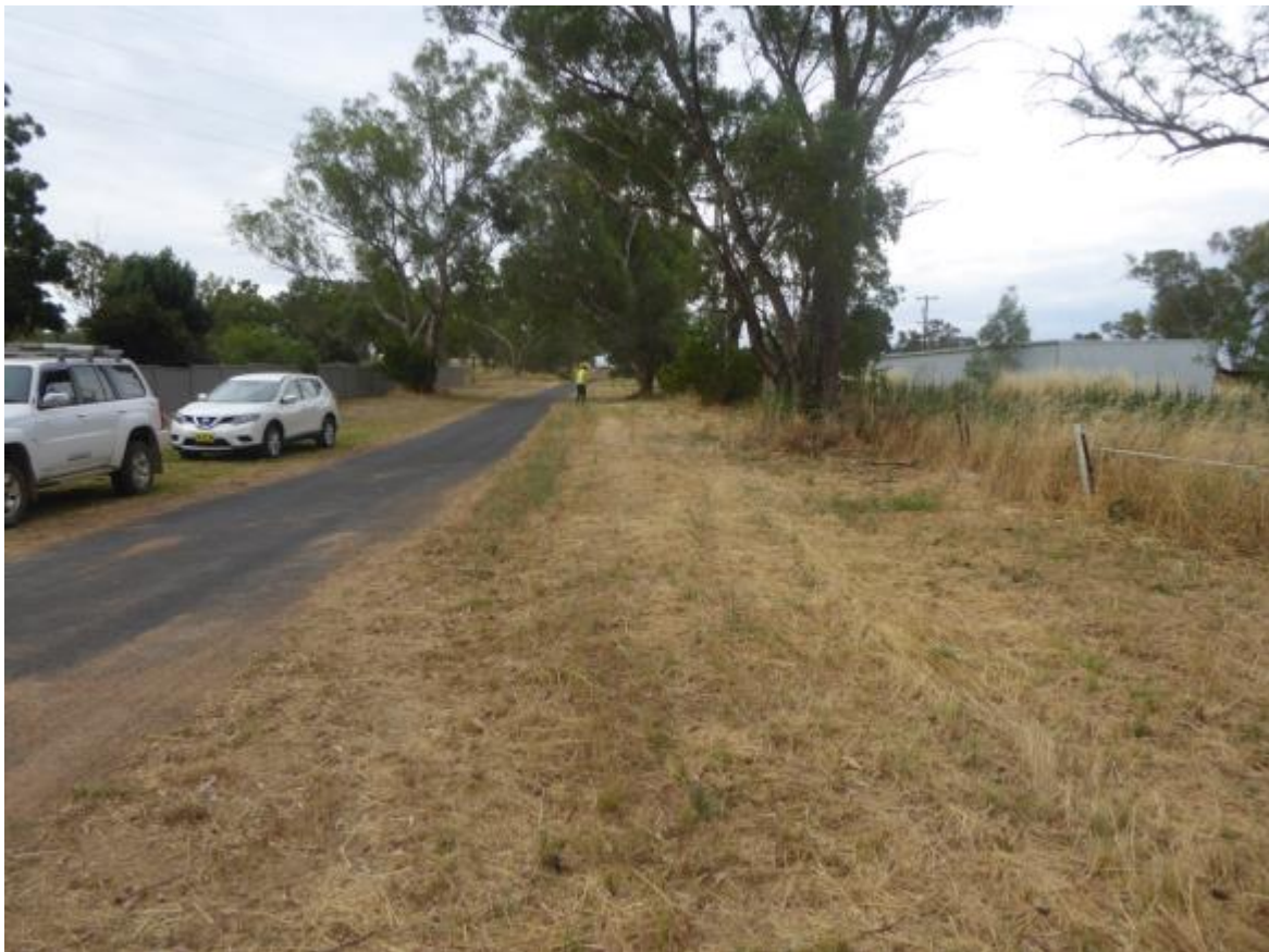
PLATE 12: Line 6A – View of the alignment, looking north from the vicinity of the intersection of Avon Road and Bournewood Road.
