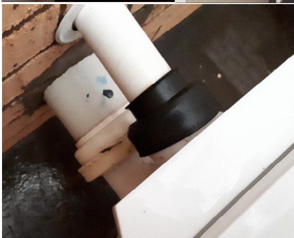
MOLONG RECREATION GROUND TOILET BLOCK - FEMALE AMENITIES
