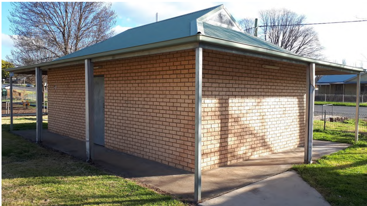
MOLONG RECREATION GROUND TOILET BLOCK EXTERNALS
