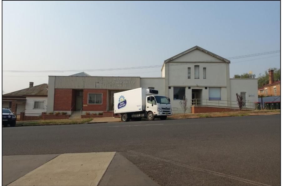
Figure 3: View of the existing buildings from the northern side of Bank Street, looking south.
