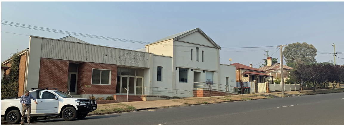
Figure 22 View of the former Arts Hall and Supper Room from Bank Street. Courtesy Architects King + Campbell PL.
