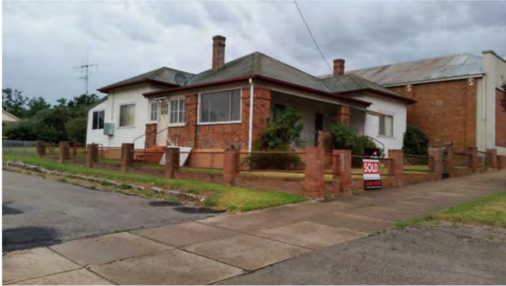
Photo 1: North-east corner of residence and part of the Community Hall extension beyond.
