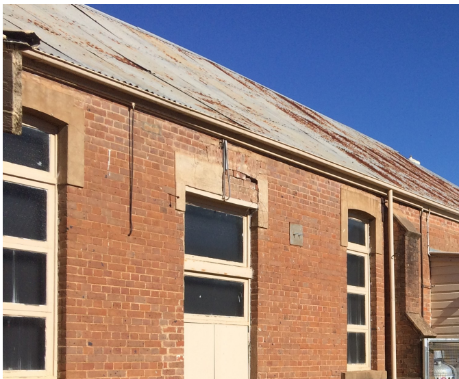
Figure 15 English Bond Brickwork with rendered heads and a stepped attached buttress. Windows have horizontal panes so were possibly replaced in the late 1930s. Image courtesy Architects King + Campbell
