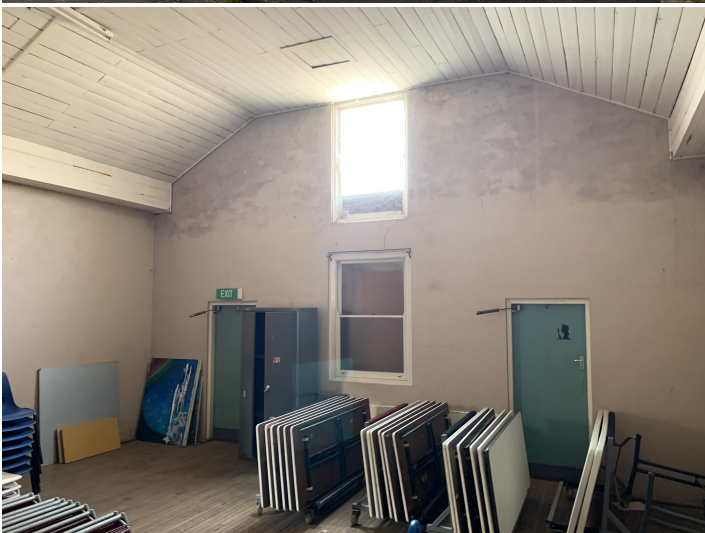
Figure 17 Signs of falling damp. Courtesy architects King + Campbell.
