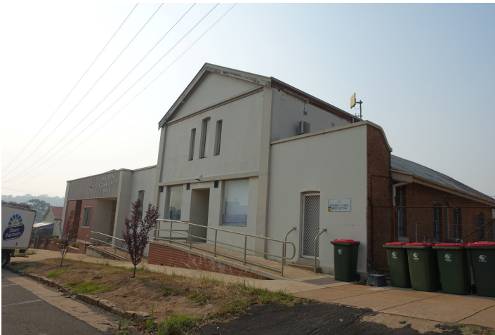
Figure 16 A fully rendered façade today. Photo Courtesy architects King + Campbell
