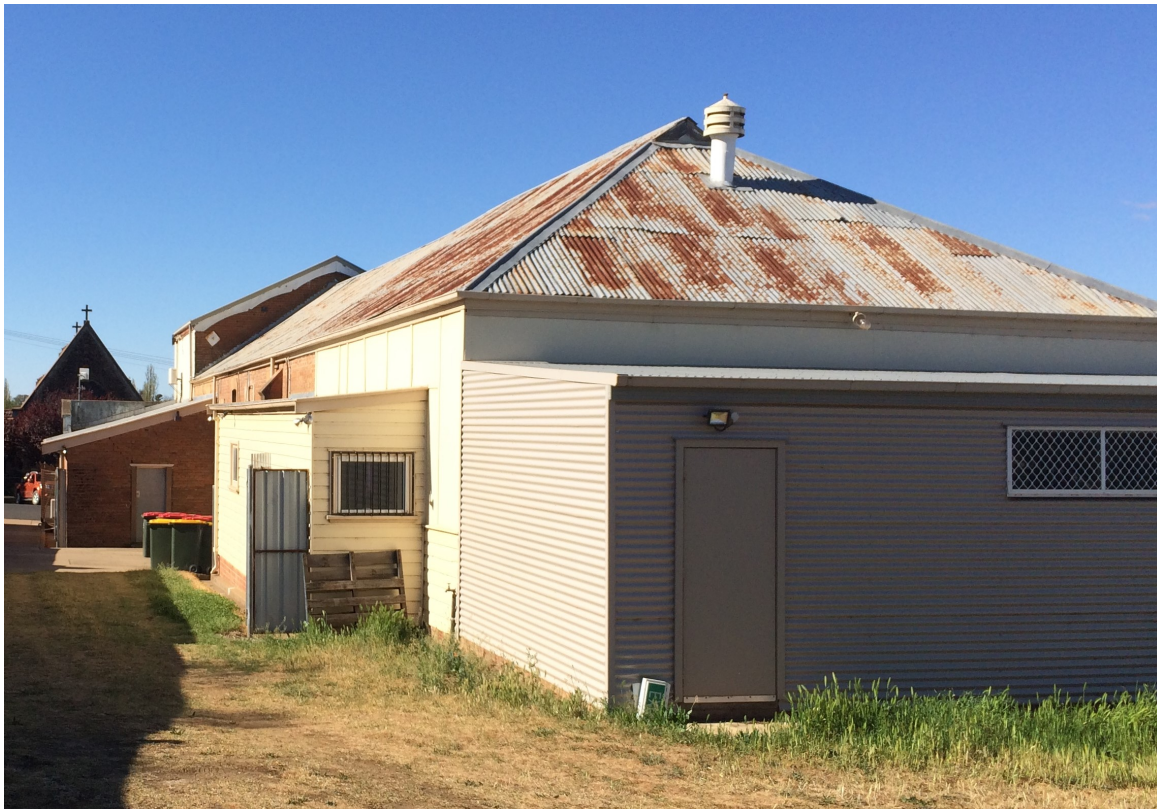
Figure 18 This rear view of the hall shows at least six stages of construction.
