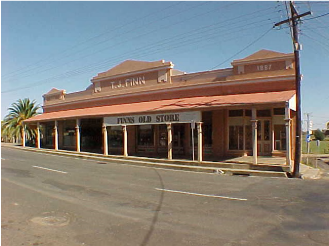
T.J. Finn's Store, Gaskill Street, Canowindra (note inappropriate signage)
