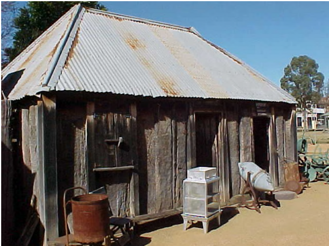
19 th century slab-walled Merriganowry Hut, relocated to Canowindra Museum. Note items of domestic technology near door: washing machine and meat safe.
