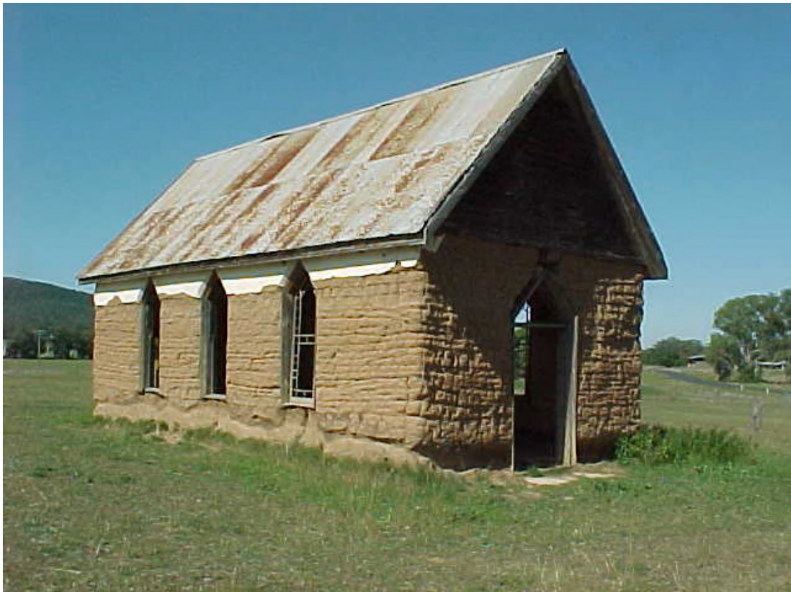
Pise (earth) walled church on Eugowra-Gooloogong road.
