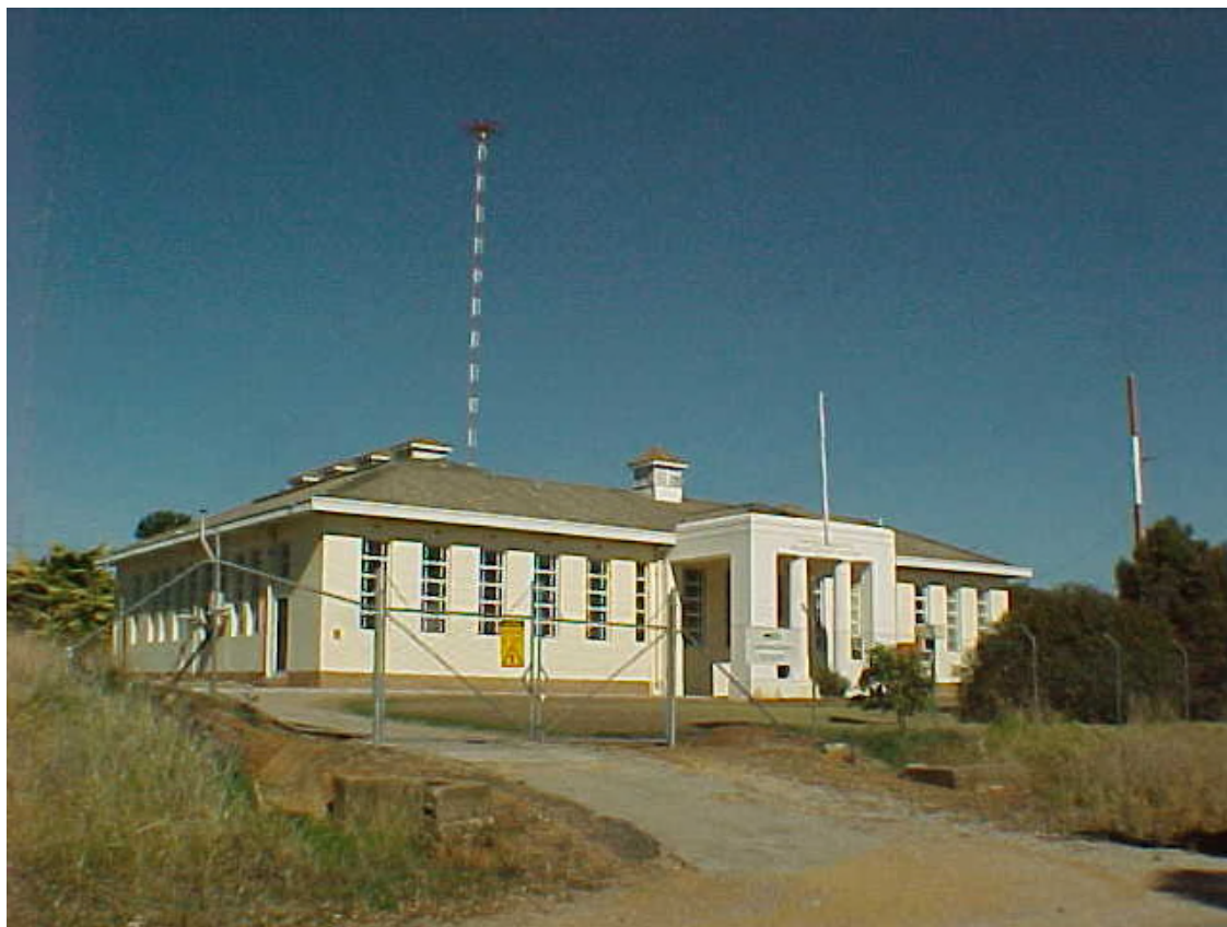
2CR (Central Regional) radio transmitter and aerial, near Cumnock
