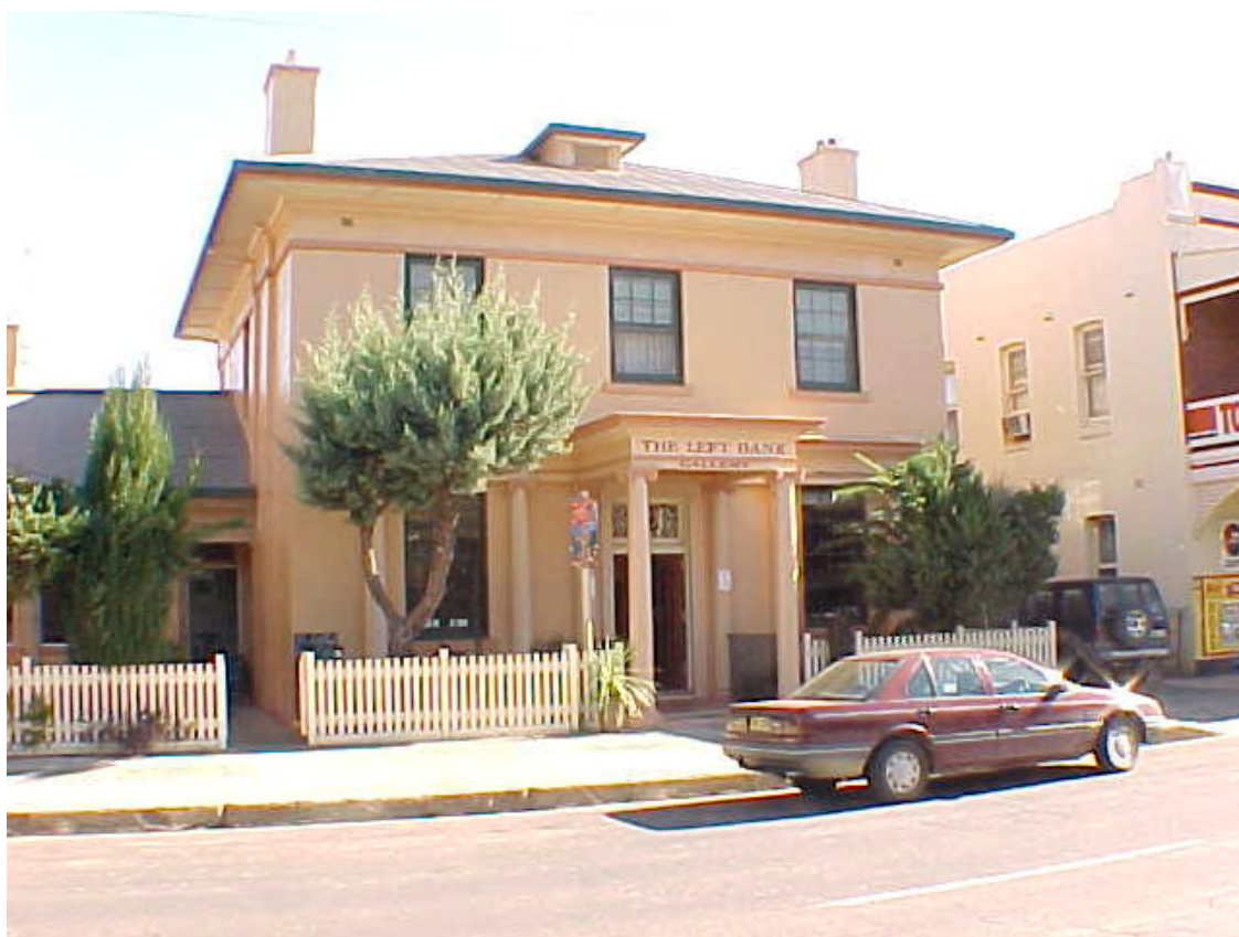
Bank of New South Wales (Westpac), Canowindra. Hardy Wilson, architect
