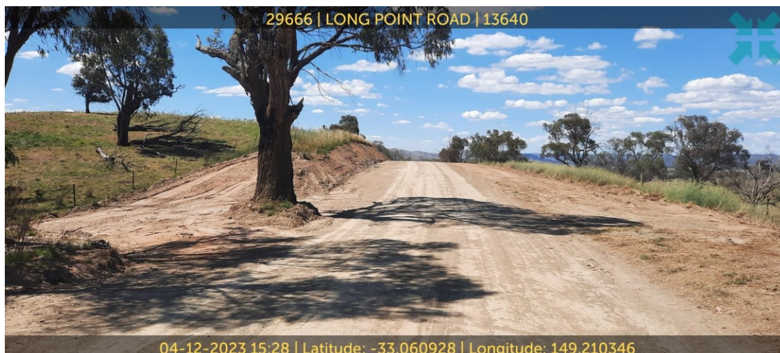
Long Point Road – Completed Works
