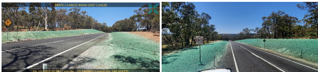
Cargo Road – December 2023
