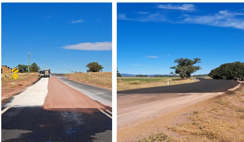
Photos of heavy patching works on Warraderry Way as they progressed from stabilising to sealing
