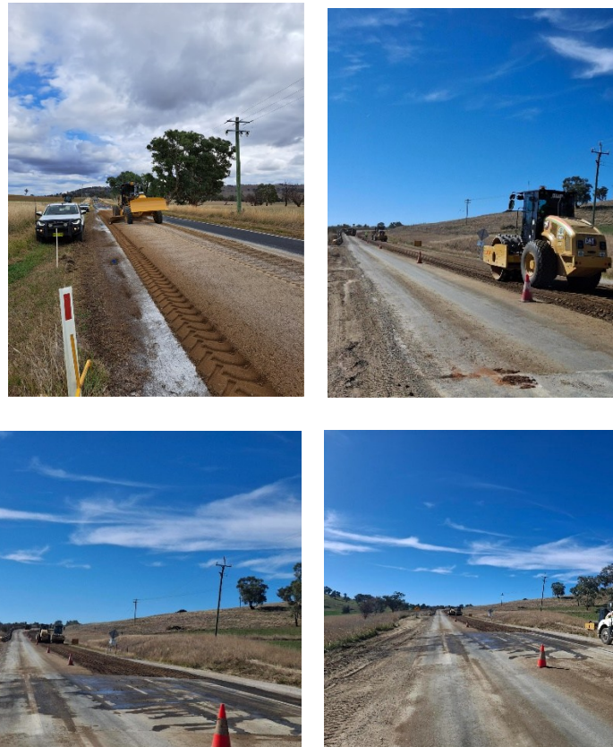
Heavy Patching under way on The Escort Way
