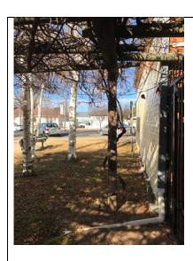
Downpipe from adjoining Yarn Market building is not connected to storm water and appears to be piped directly onto the ground within the Village Green
