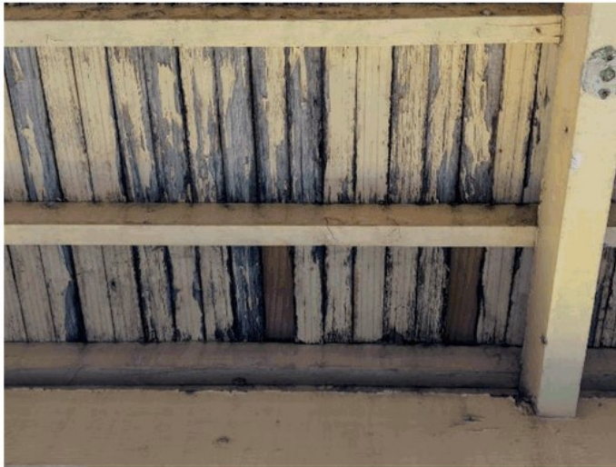
View of damaged floorboards
