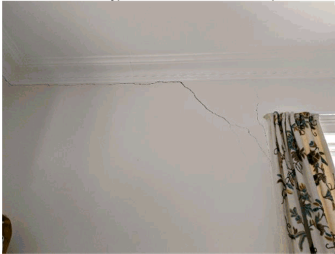
Photo 3 A typical crack in the vicinity of the window at the front northern corner. The verandah has also subsided external to this area.
