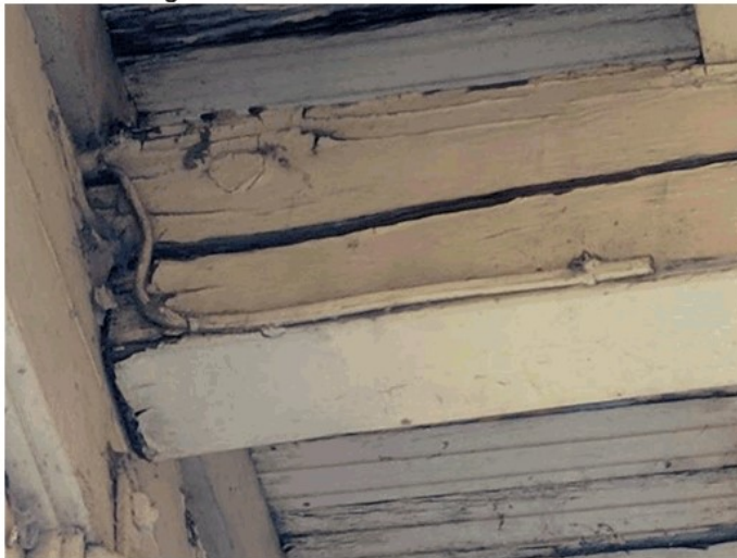
View of a damaged bearer and redundant electrical cabling.
