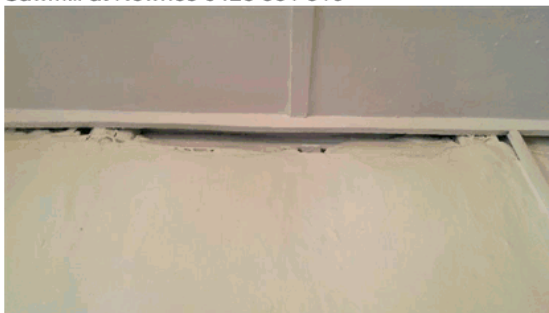
Photo 5 A typical internal view of the ceilings which consist of metal sheets and timber battens over the junctions.
