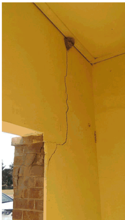
Figure 6 Corresponding entry cracks
