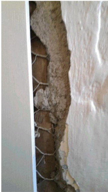
Photo 6 A typical wall detail, exposing the timber post wall, wire mesh and plaster. This is a variation of the wattle and daub where the local timber has been used in conjunction with fencing wire and lime based plaster. The early decoration is also something to consider – these can often be expressed using small framed panels on the walls.
