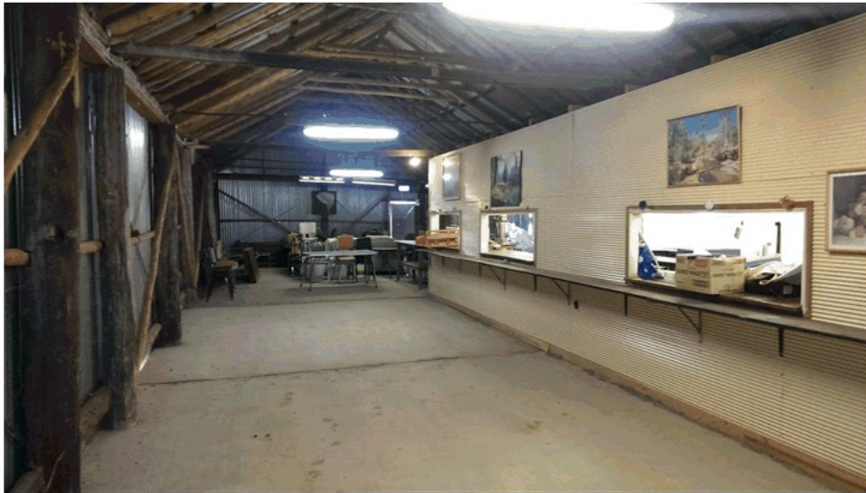
Figure 3 New mini-orb wall cladding around the kitchen
