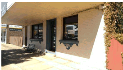
Photograph 15 Street elevation. The rendered decorative dressings under the window sills – originally these were Pale Cream and the window sills strong red.
