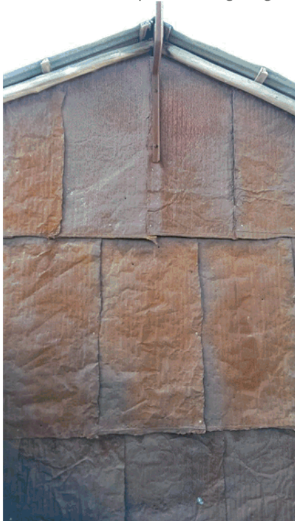
Photo 10 A rare cladding using flattened oil drums.
