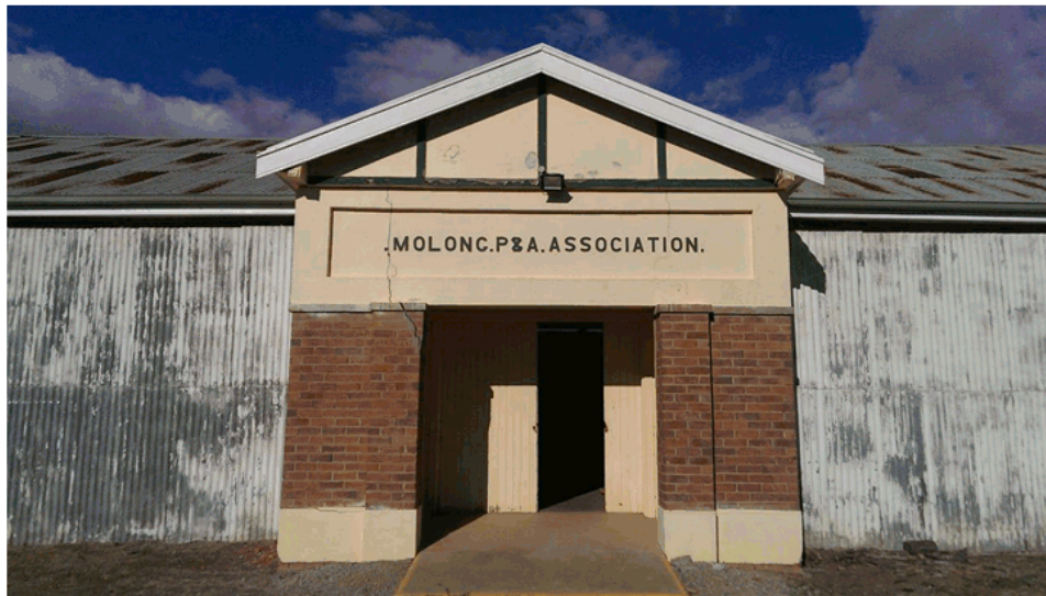
Figure 5 View of the rusted roofing sheets and the damaged entry
