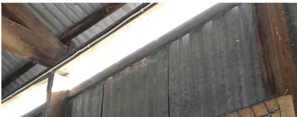
Figure 8 View of the natural ventilation gap.
