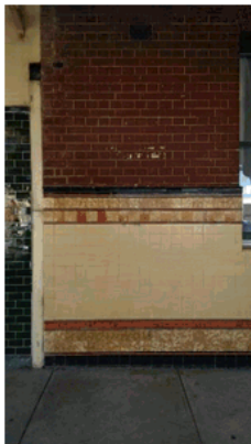
Photograph 37 Option one is on the brickwork above the tile line. This is too high and affects original brickwork.
