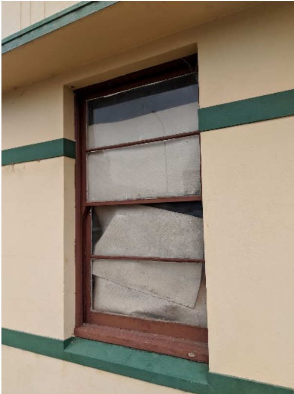
Photo 2 An original window to be retained and restored
