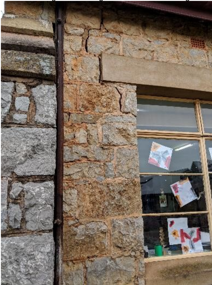
Photograph 16 Engineers to review lintel and stonework – asap.
