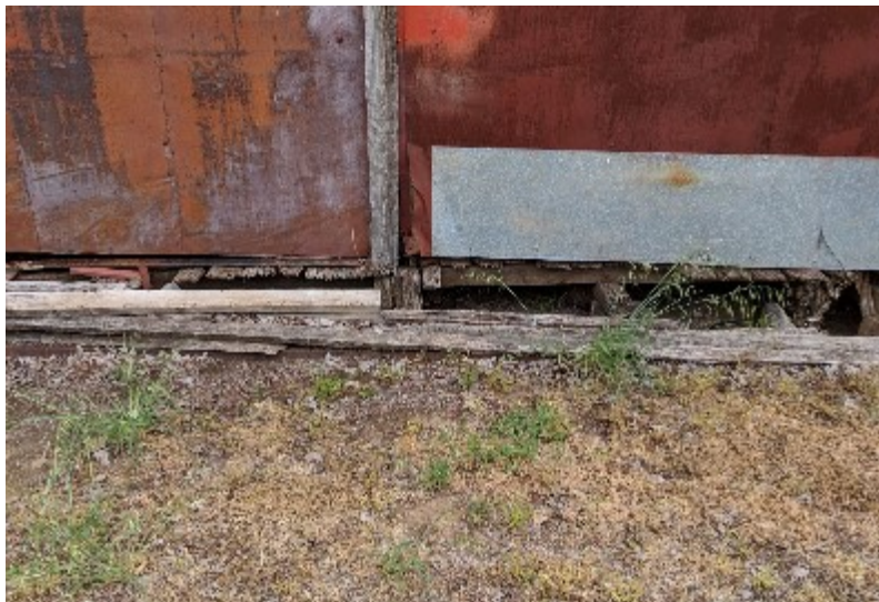
Photo 10 Proximity to the ground has caused extreme decay.
