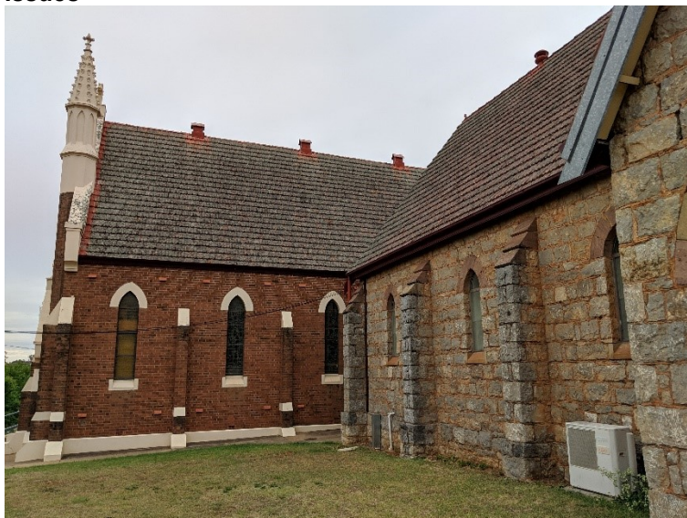
Photograph 1 A detail view of the two church buildings and their replacement Marseille pattern terra cotta tile roofs
