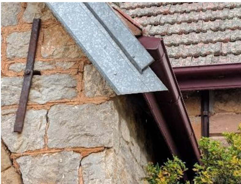
Photograph 8 Early steel 'rod and stick' bracing systems are evident on both the porch and the end wall. These should be reviewed by the Consulting Engineers as they may no longer be effective and may lead to consequential damage. The galvanised steel flashings replacing or covering the traditional barge boards detract from the traditional details and heritage significance.
