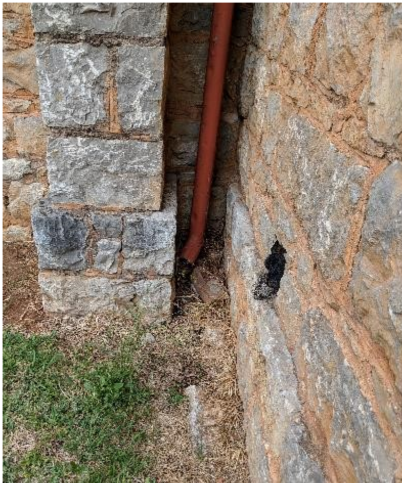
Photograph 6 Downpipes which discharge on to the ground around the building lead to foundation movement and rising salt damp. All stormwater should be piped to the street or
