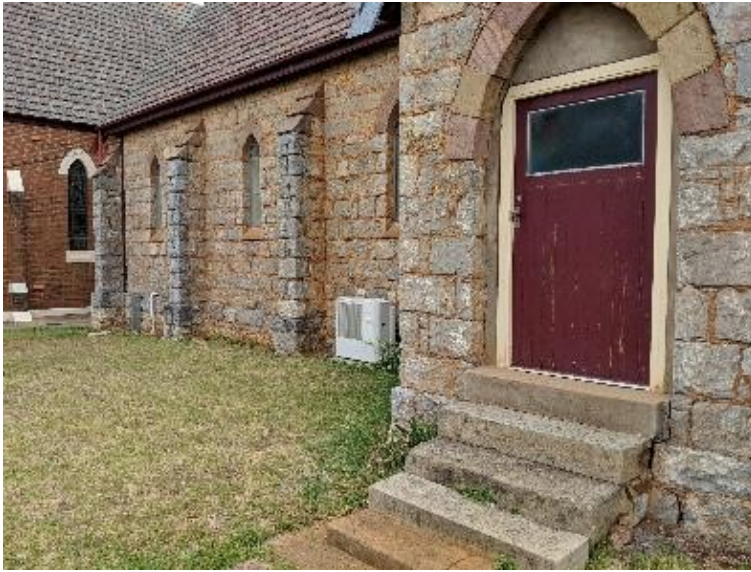
Photograph 7 The perimeter of the building has grass and planting adjoining the four stone walls and this leads to foundation movement caused by uneven drainage. The door infill detracts from the character, appearance and significance of the Elevation. Restoration of the opening is recommended.
