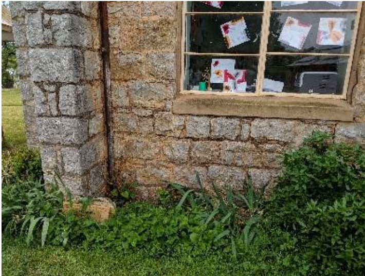
Photograph 15 Engineers to review the effectiveness of the bracing, the lintels and stone repairs using Helifix or similar in order that the wall be reconstructed to act as a composite element without the point loads exerted.
