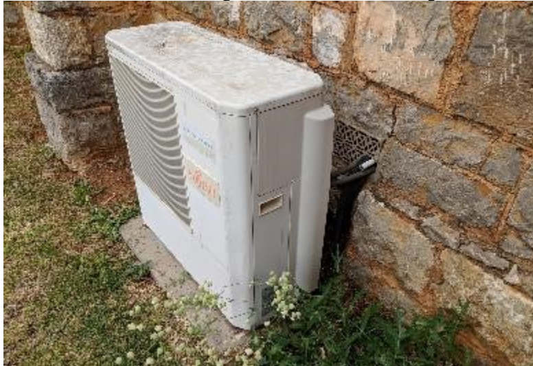
Photograph 5 An example of an external compressor for split system air-conditioning system: the installation of services which detract from the character and appearance and hence heritage significance of the site and building.
