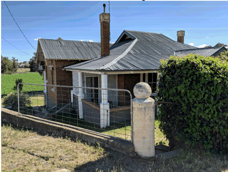
Photo 4 The adjoining property to the NW boundary. Brick and iron traditional dwelling set low on the site. No existing boundary planting to the adjoining boundary. Screen hedge planting along the front boundary.
