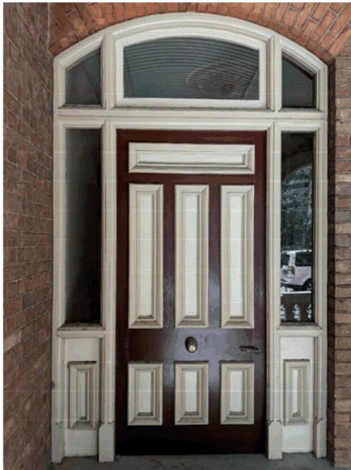
Door example in similar coloured brick walls, noting the brick header course
