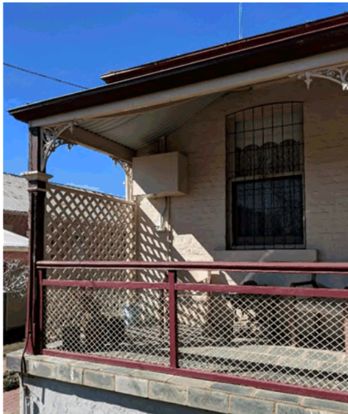
Photograph 1 View of the front corner.
