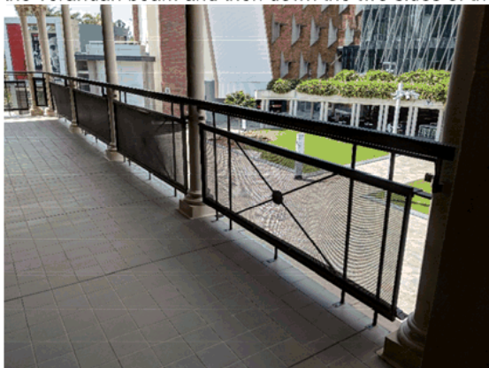
Photo 1 The purpose of the following three photos is to illustrate the alternative for a balustrade which uses perforated wire sheet as the infill. When viewed from front on it is almost invisible.
