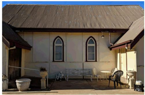
The side elevation next to the entry drive. The brown roof is not appropriate and Shale Grey will match the roof to the rear. Note that some glass panes have been damaged and replaced. The following are useful contacts for replacement glass which is appropriate in the traditional windows:
