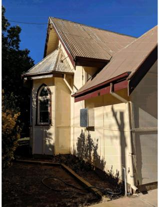
The front elevation noting the bay window and use of the Red and Cream. The joinery is to be restored. Elements of damaged fibro need to be replaced in compliance with WorkCover practice and the associated new cover battens.
