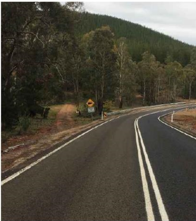
Four Mile Creek Road upgrade
