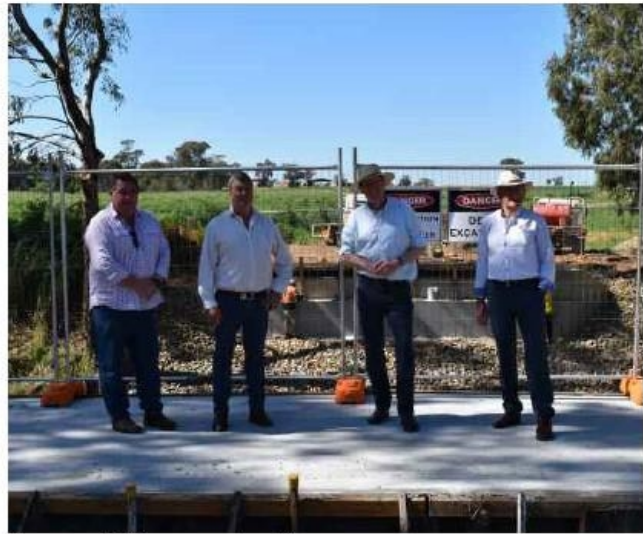
Bangaroo Bridge reconstruction
