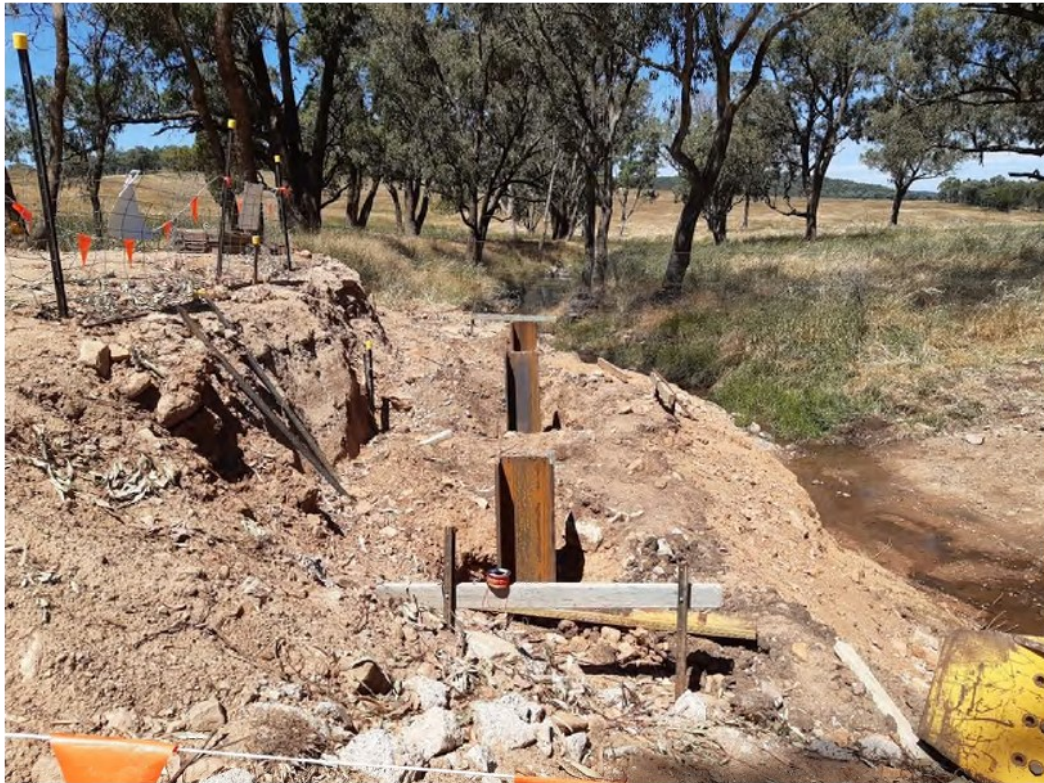
Driving piles in progress
