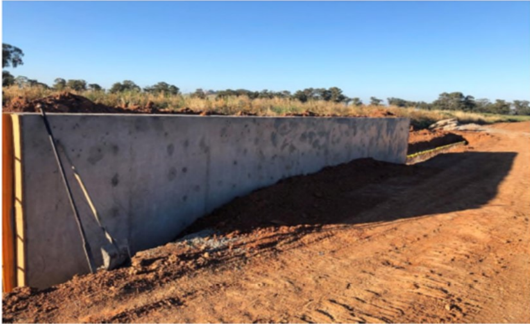
Exposed finish of Showground retaining wall
