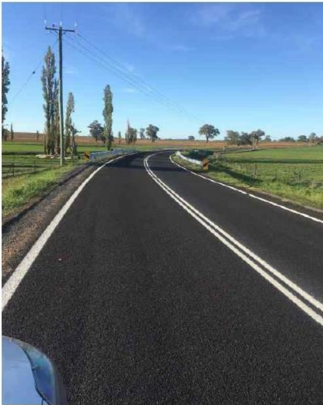
Davy's Plains Road upgrade
