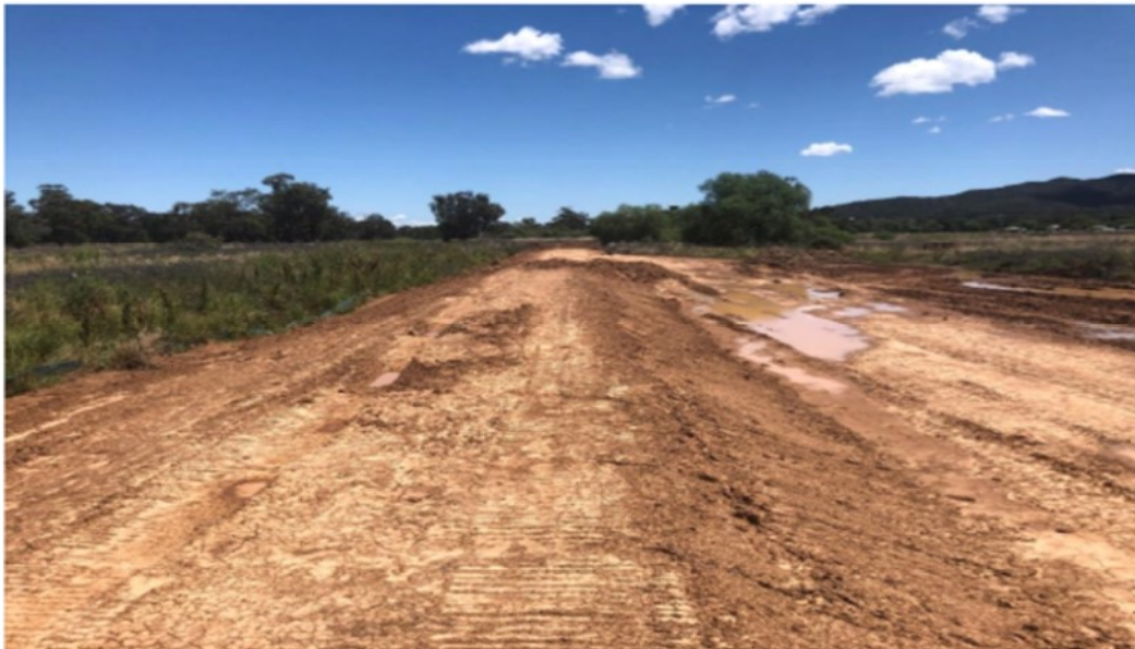
Levee core placed, awaiting capping layer
