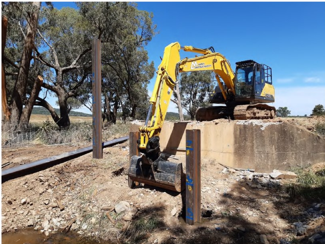
Demolition works in progress
