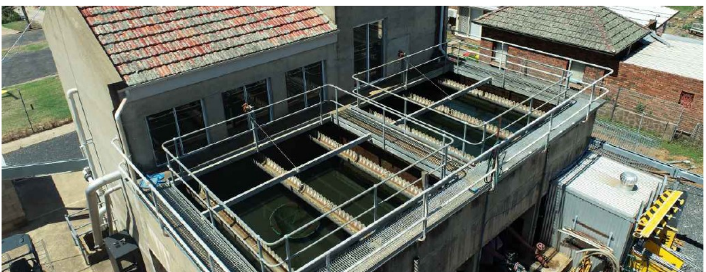
Cabonne Council Water Treatment Plant - Molong
