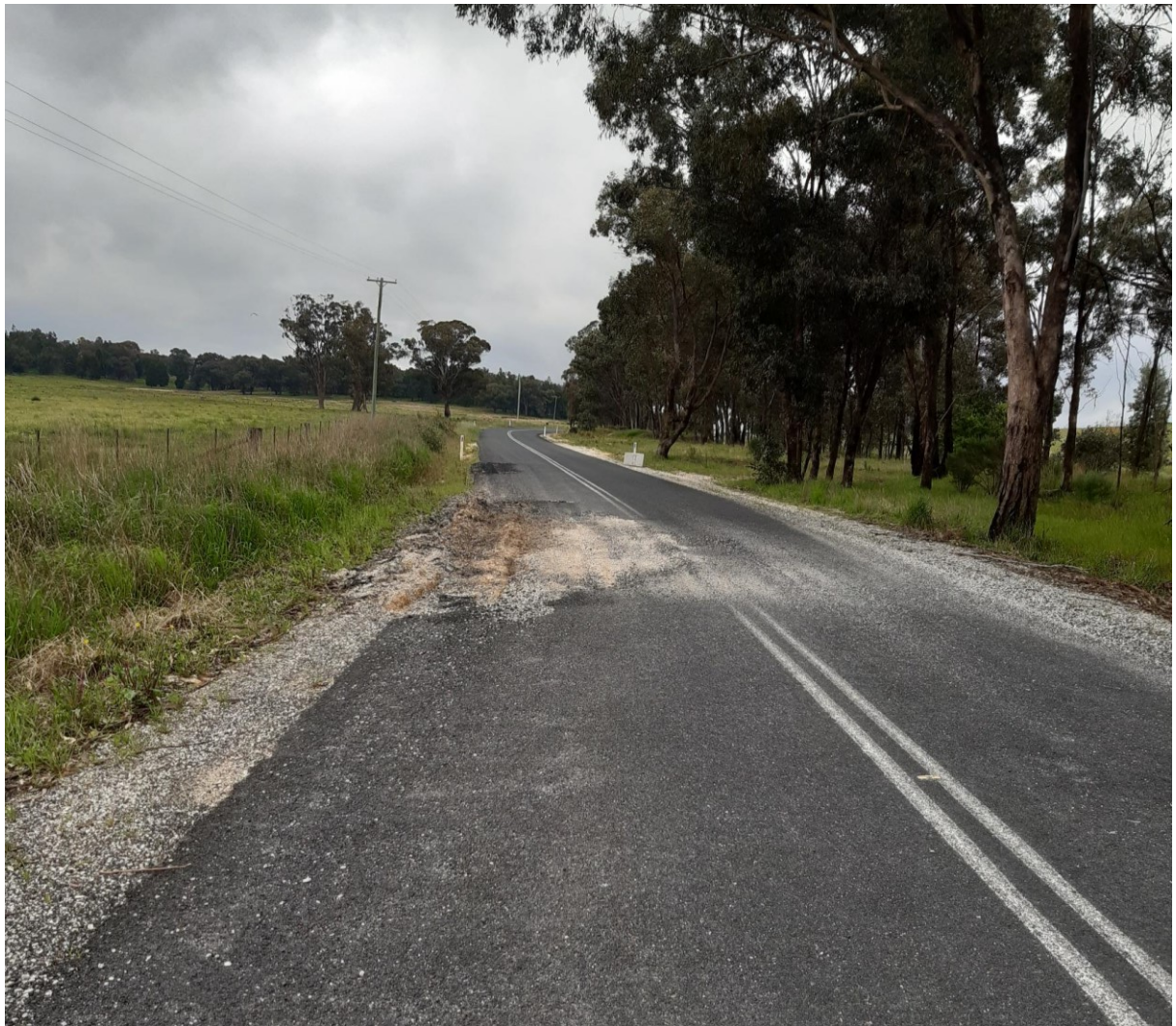
Photo of Bocobra Road, damage from spring to sealed road
