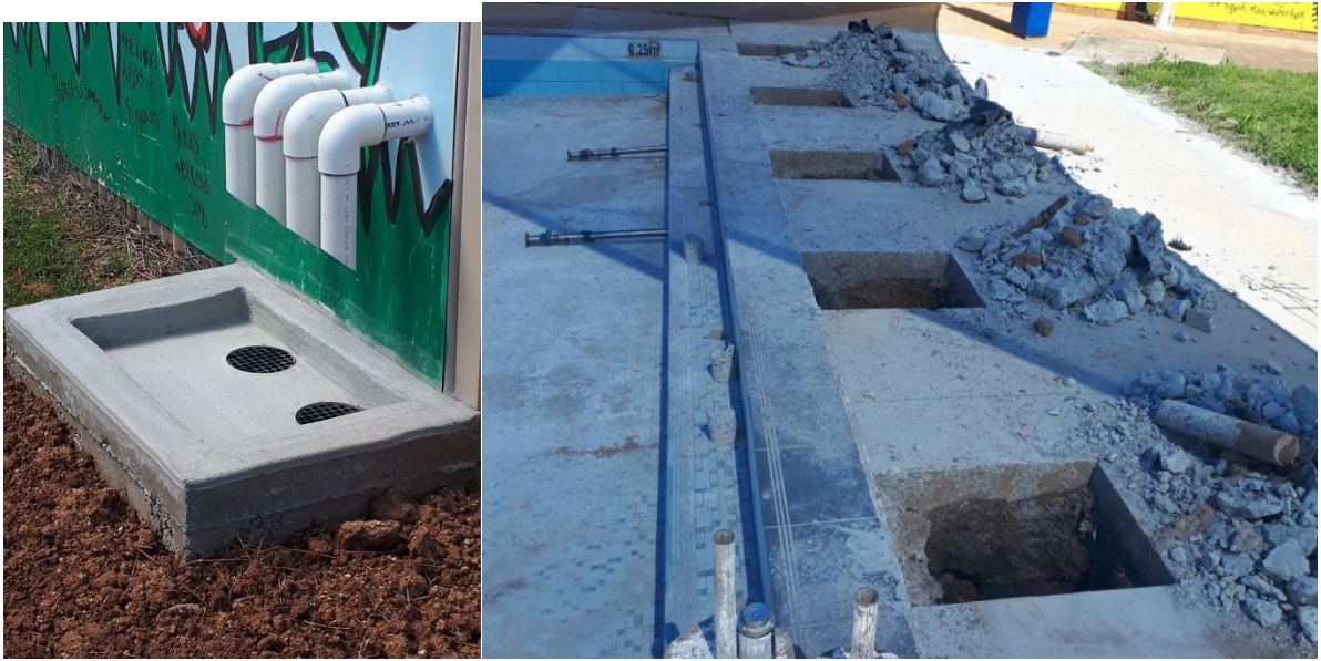
Back wash – new connection, subsurface piping locating – Eugowra Pool
