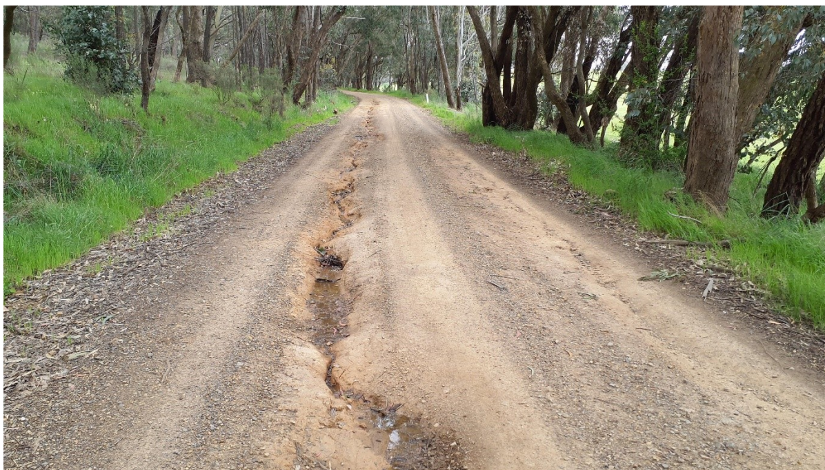
Photo of Long Swamp Road, longitudinal scouring following rain event
