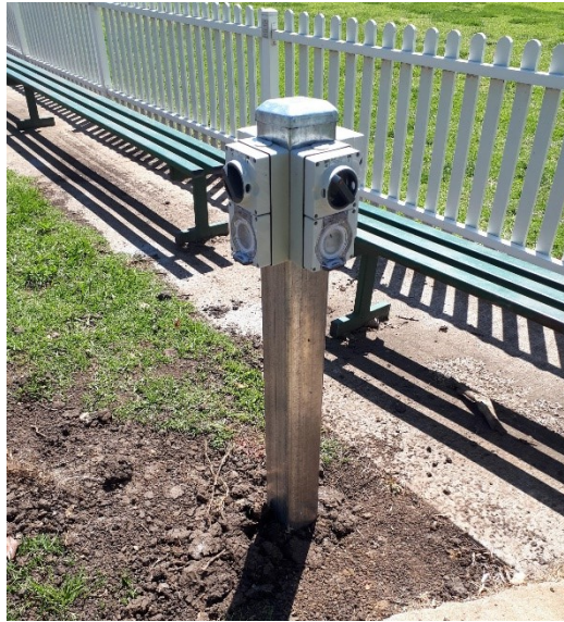
Power Bollards – at Molong Rec Ground
