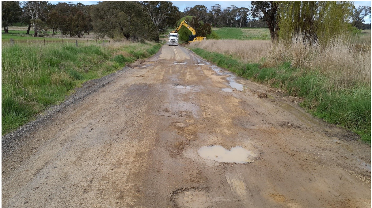
Photo of Spring Hill Road, damage from spring to sealed road
