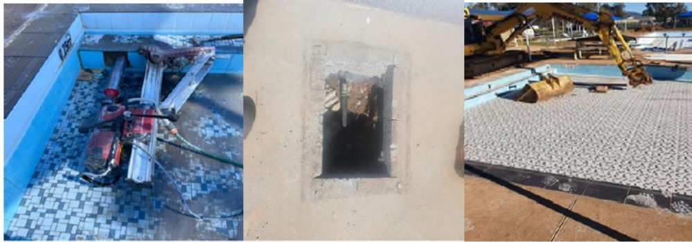
Core drilling, subsurface piping locating – Eugowra Pool
