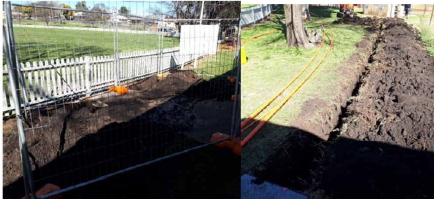
Service Trenching work – commenced at Molong Rec Ground
