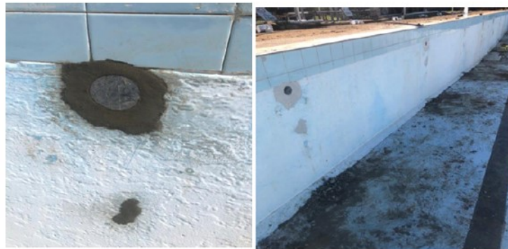
Internal pool interconnections completed – Manildra Pool
