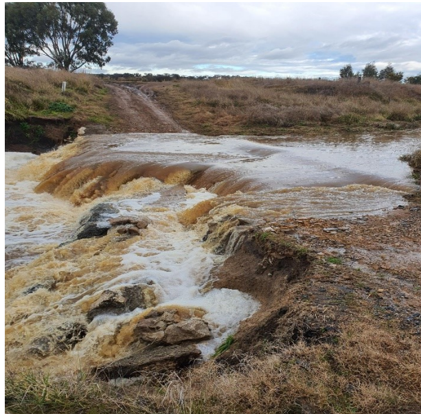
Burrawong Road culvert washout
