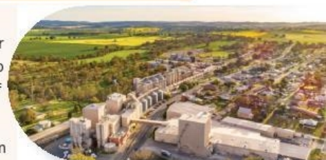
Manildra Mill, Central West NSW.
