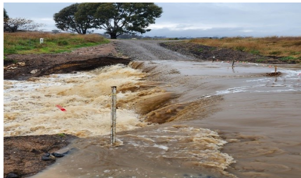
Burrawong Road culvert washout
