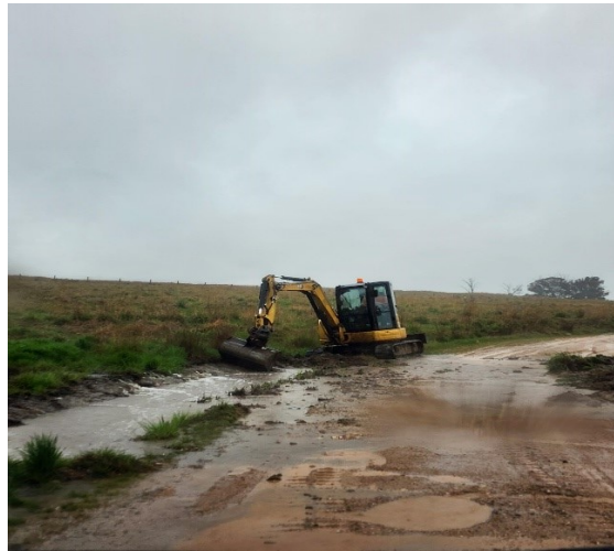
Opening up the drains on Burgoon Lane
