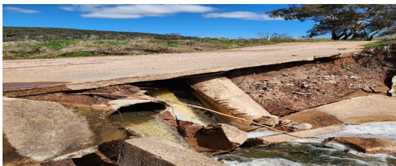
Causeway washout on Pinecliffe Road
