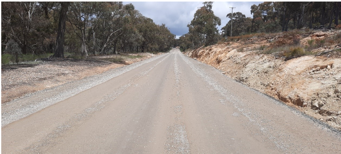
Post-stabilising – Burrendong Way
