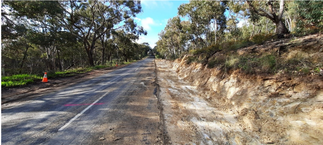
Boxed out drain & road shoulder – Burrendong Way
