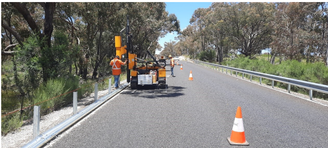
Installing Guardrail – Burrendong Way
