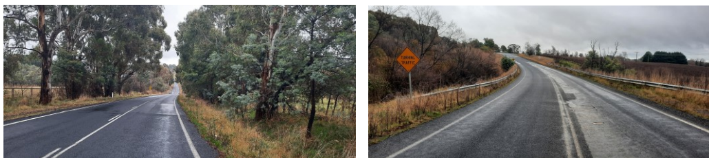
Cargo Road – Before Work was undertaken
