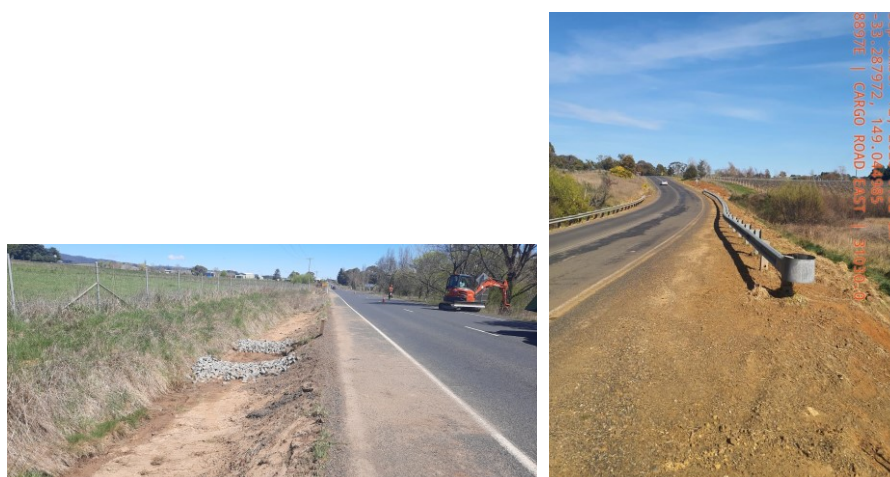
Cargo Road - Completed
