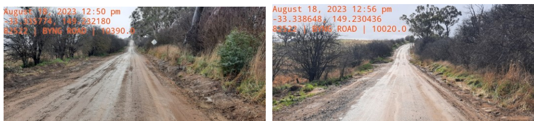
Byng Road - Completed
