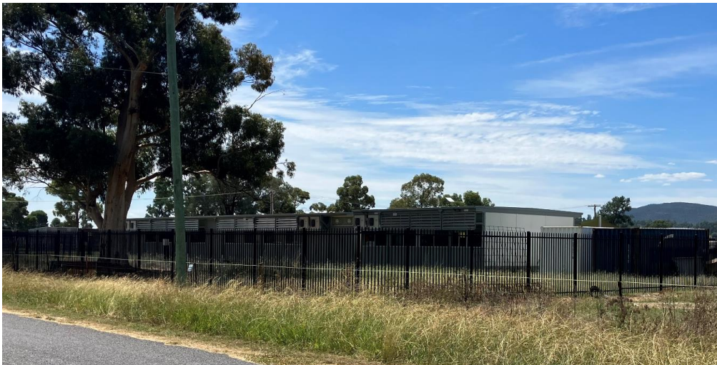
Temporary site of pre school
