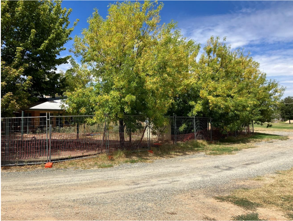
Flood damaged former pre school site
