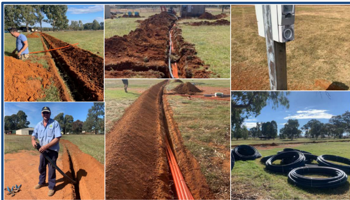
Figure 14 – Power and water supply Power and water supply was improved at the Showground during Stage 1 works, Cudal Village Masterplan 2021.
