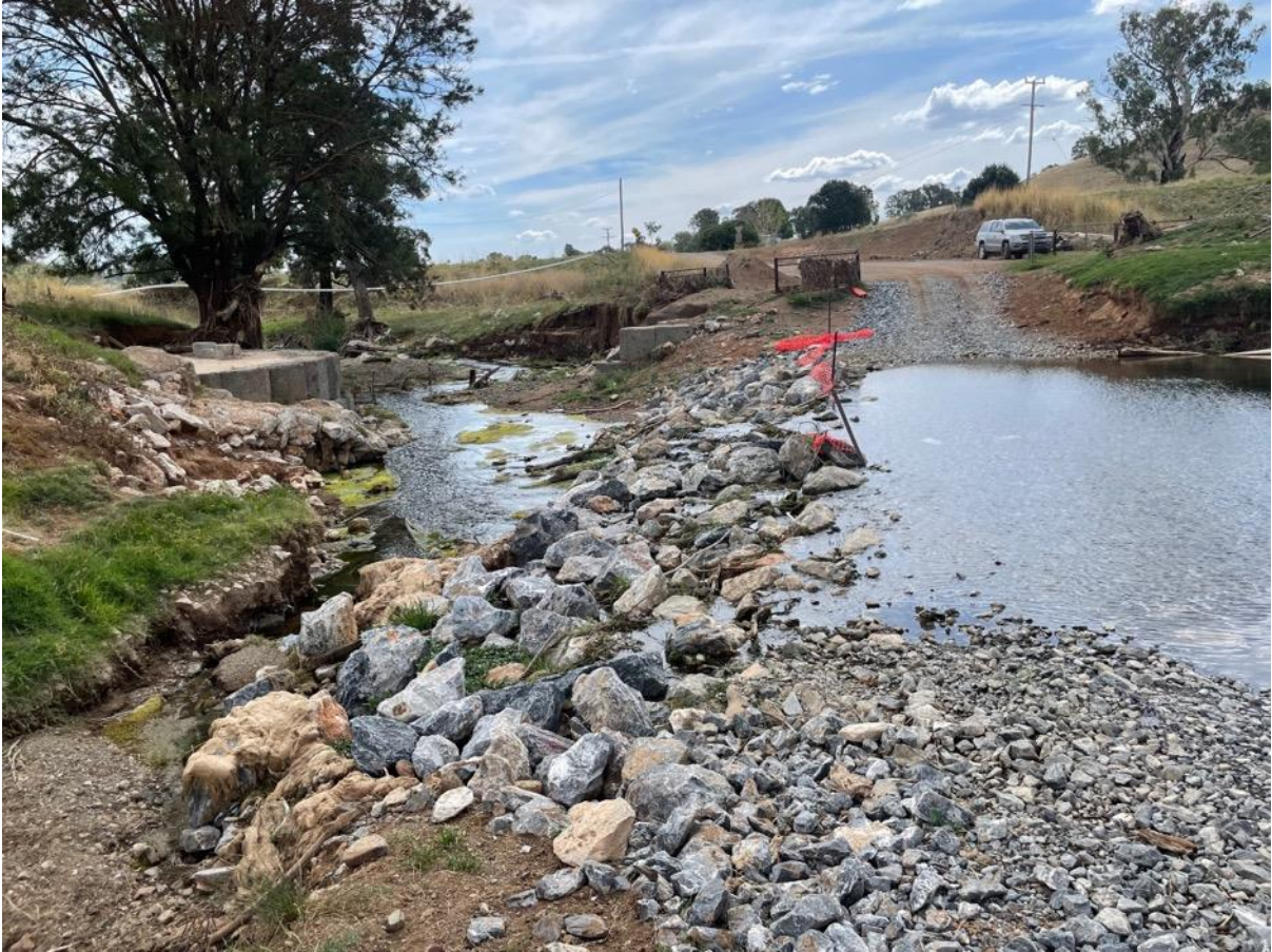
Figure 4 Temporary Causeway (right) and Remains of Bridge (left) looking North
