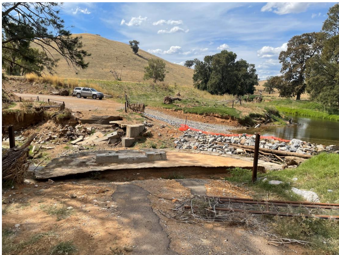
Figure 5 Remains of abutments
