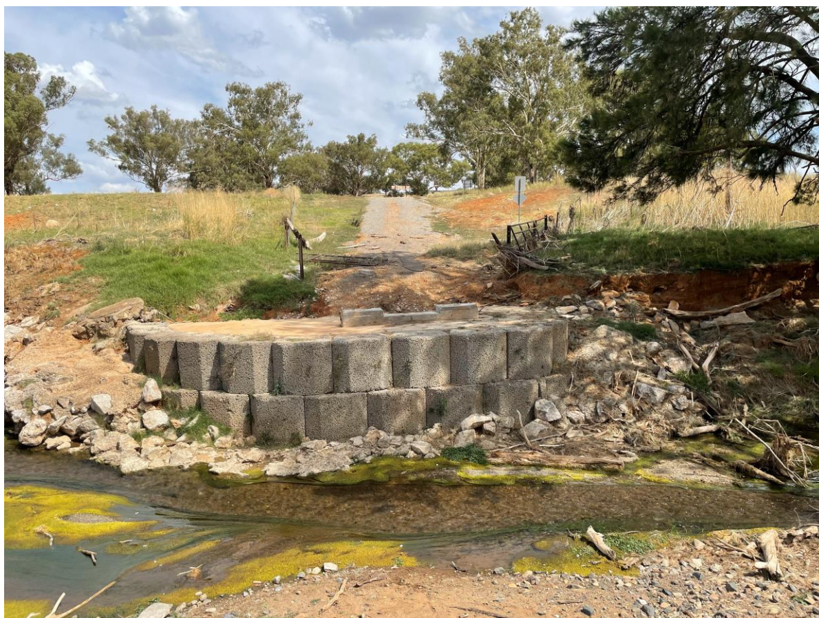
Figure 6 Southern Abutment remains somewhat in tact
