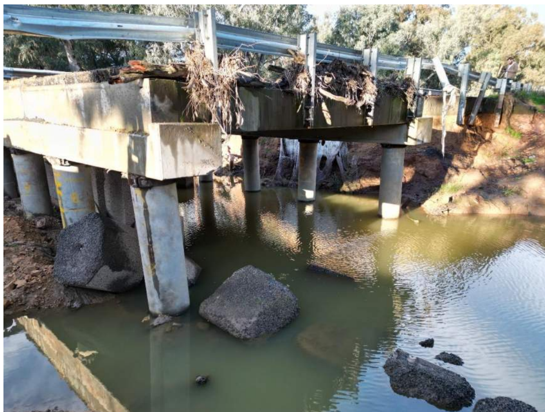
Figure 5 Concrete Block temporary abutment protection washed away.
