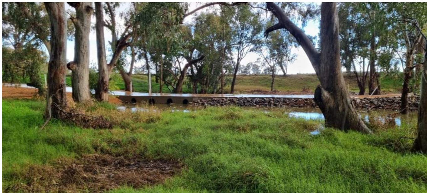
Figure 4 Temporary culvert-causeway sidetrack downstream from bridge
