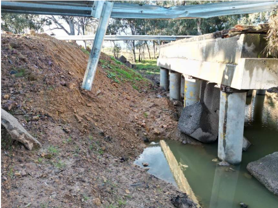
Figure 6 Significant Scour Behind abutments
