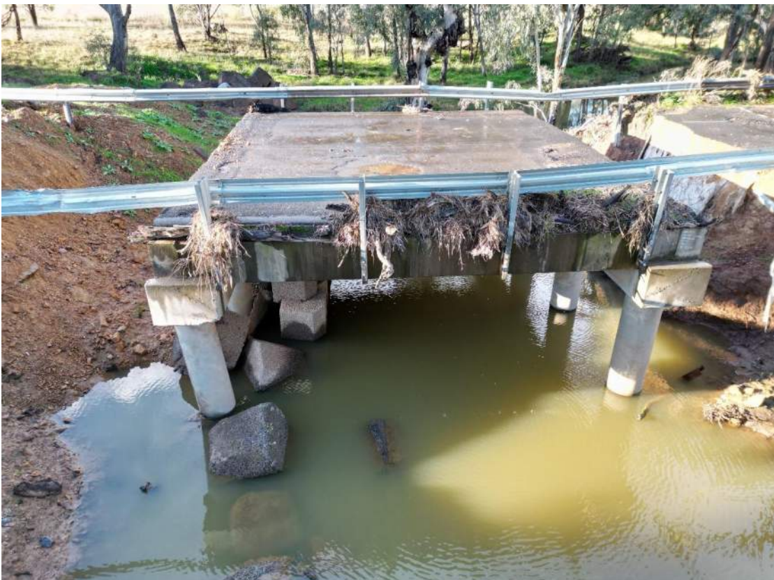
Figure 7 Looking upstream, significant debris evident.
