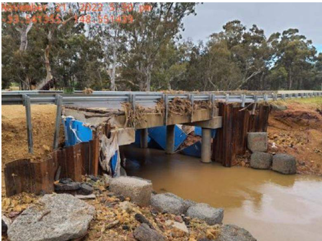
Figure 1 Temporary Repair of Bridge in 2022
