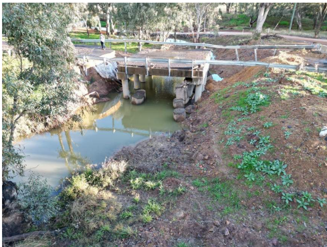
Figure 3 View from Upstream of existing bridge with washed away approaches.
