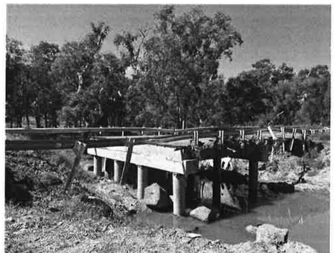
Photo 4 Remaining concrete strucutree of Nyrang Bridge with approaches washeded away
