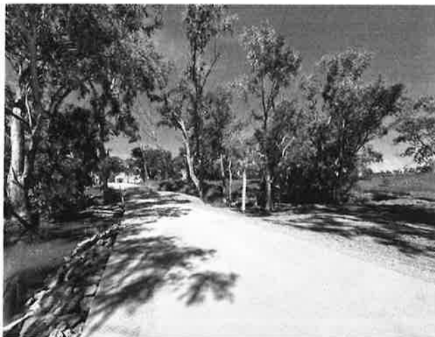
Photo 3 Unsealed tempoary culvert-causeway sidetrack downstream of Nyrang Creek Bridge
