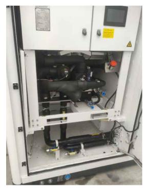
figure 12-6 Removal of liquid-cooled unit front baffle
