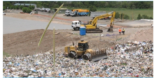
Once garbage is placed inside the landfill cell, a layer of soil is added on top to help reduce the smell, litter and interaction with pests.
