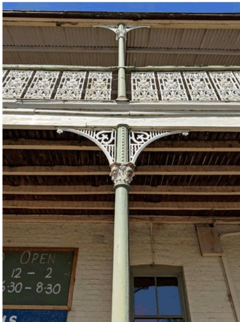
Figure 5 The third column in from the left hand end. Alignment is good and timber in place.
