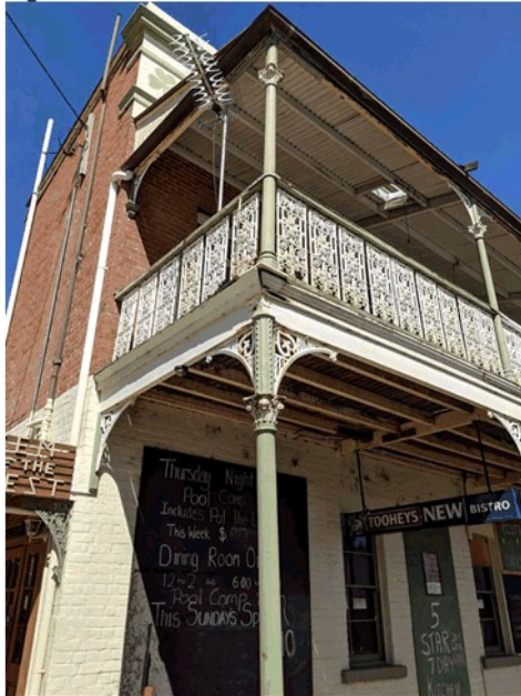
Figure 8 The corner cast iron column and damaged timbers at the first floor junction
