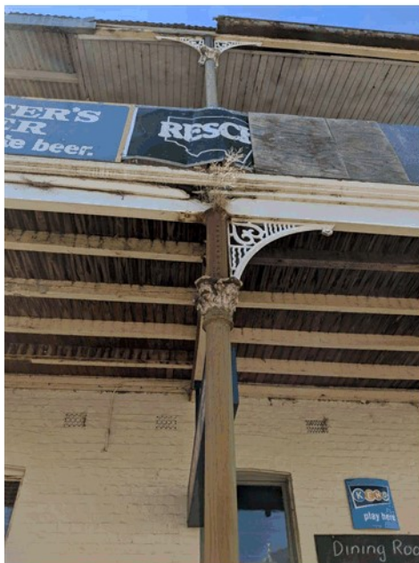
Figure 2 The next column from the SE corner, noting the rotted junction at the floor and loss of gutter at the roof.
