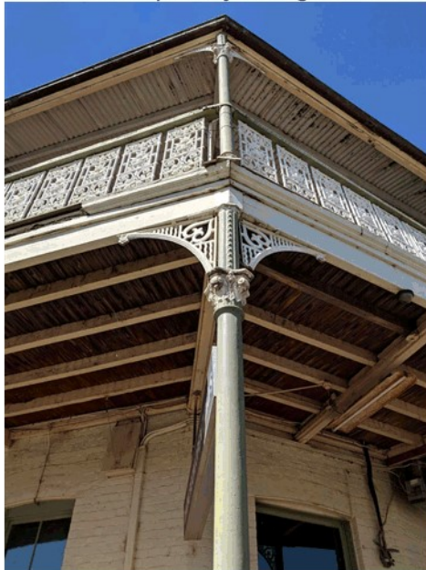
Figure 4 The corner, noting the loss of timber moulds at the floor level and lack of downpipes.
