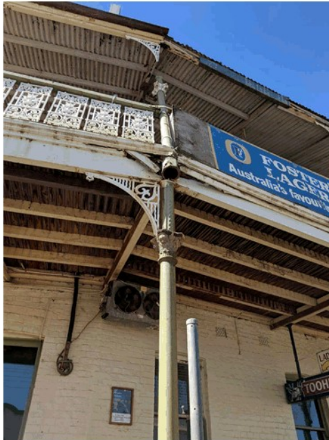
Figure 3 The column which has given way and the missing gutter above. The handrail ties are possibly holding the column in place.
