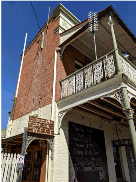
Figure 9 The end view and sole downpipe.
