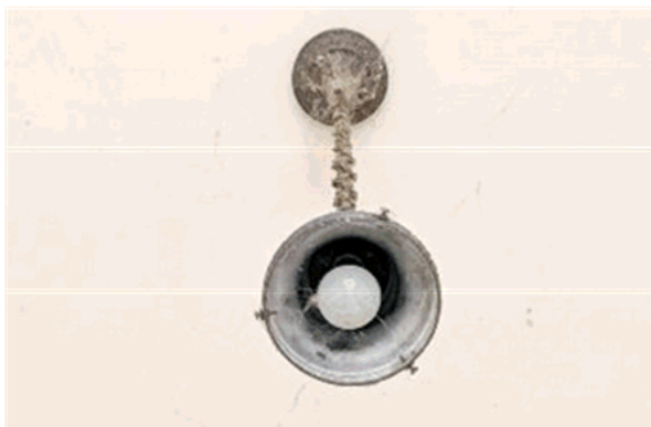
General view of the memorial foyer at the entrance, noting the missing glass to the light fitting.
