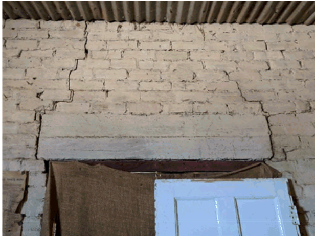
Interior view of the original skin of brickwork and lintel
