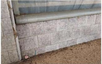
Figure 4 The ceramic tile facing and nickel shopfront - significant element. Generally intact, these finishes are intended to be weather protected and will decay rapidly is there is no verandah or awning.
