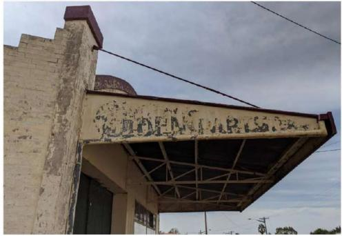
Photo 6 The side view illustrating the suspended awning and end pier with vaulted parapet.
