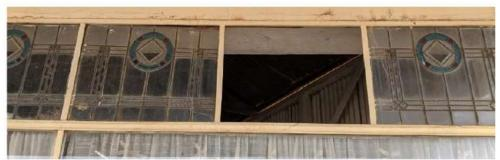
Photo 3 A detail view of the top lights or hamper panels with their leadlight and coloured glass set within a nickel frame – a significant element.
