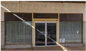
Figure 6 The full shopfront element, noting the replacement door set. The corporate branding is showing through on the painted area above the top lights.
