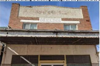
Figure 7 The full façade including the parapet detail with loose bricks, the Burgess Bros signwriting, then the garage rendered sign, the replacement aluminium windows, three suspension points, awning with minor angle framing and two end trusses - significant element. It is probable that the awning was erected with the building however a replacement awning or verandah could take either form in a simple steel construction.
