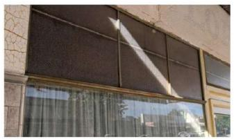
Figure 5 The upper portion of the shopfront including the nickel shopfront frame, stippled glass to the hamper panel area and special scrolled nickel details to the frame - significant element.
