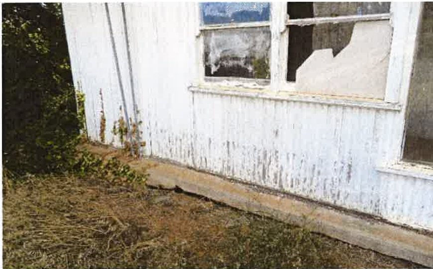
Figure 25: Detailed view of damaged cladding and timber, broken windows, gap between the ground level and concrete slab
