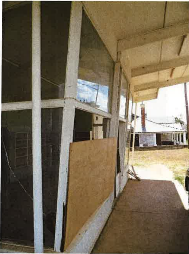
Figure 28: Detailed view of broken, boarded up windows
