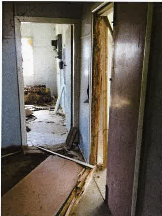
Figure 29: View of severely termite affected timber doorways
