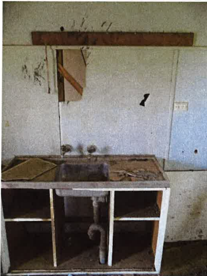
Figure 33: View of former kitchen area with walls with holes from vandal damage, theft of fittings
