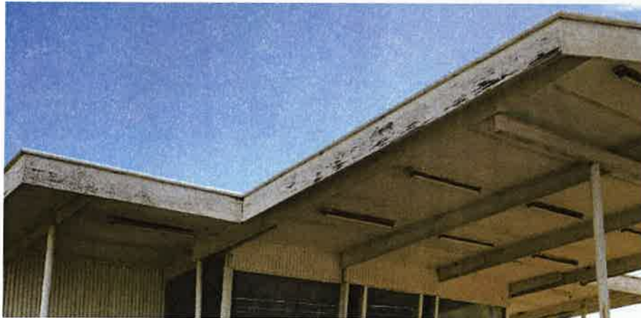
Figure 20: Detailed view of weathered and water damaged timbers
