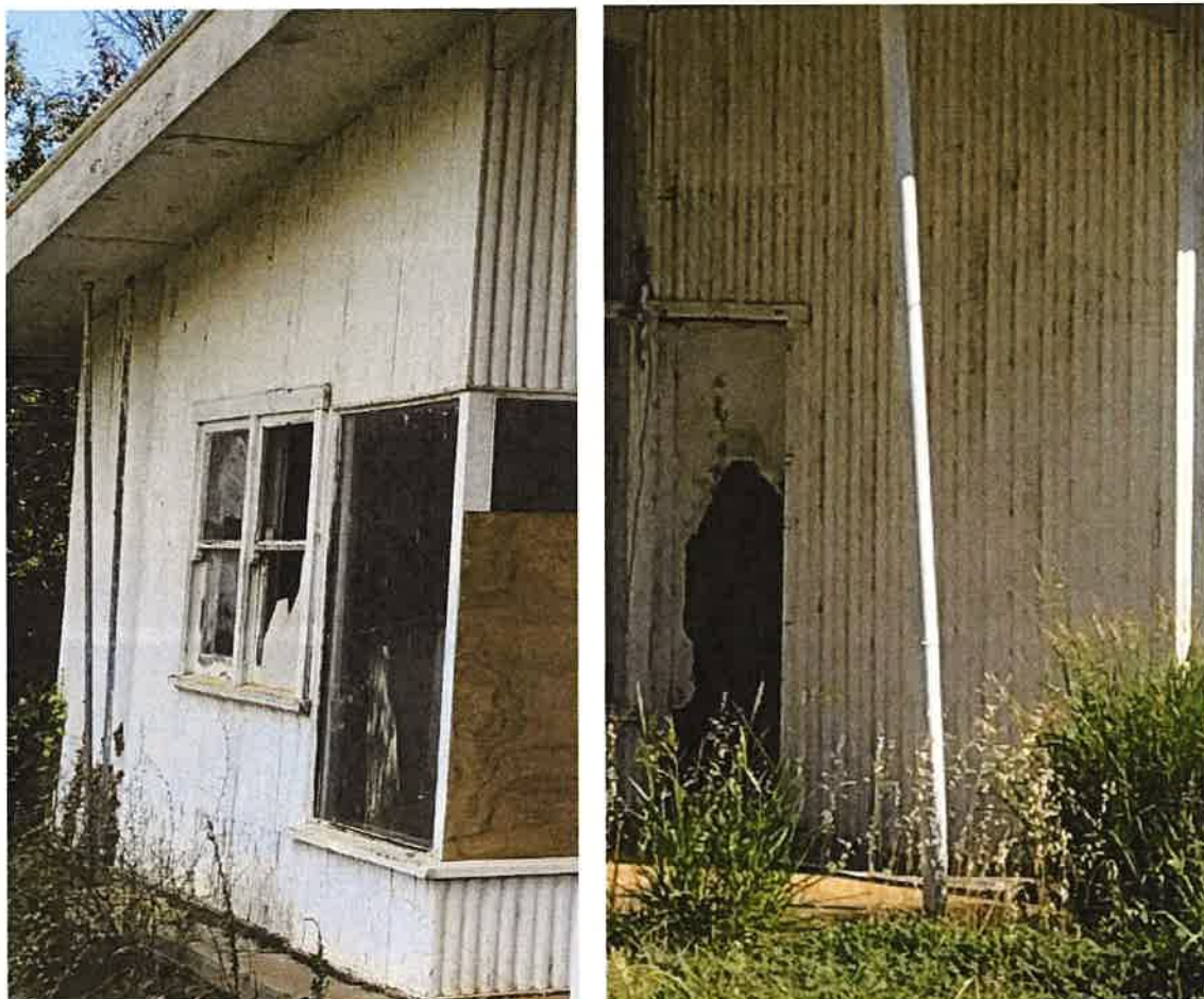
Figure 21: Detailed views of weathered and water damaged cladding
