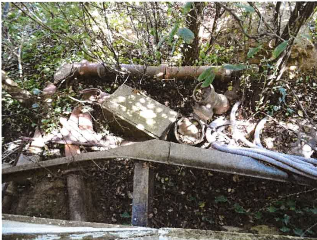
Figure 41: Environmental weeds growing out of shattered sewer piping at the rear of the building
