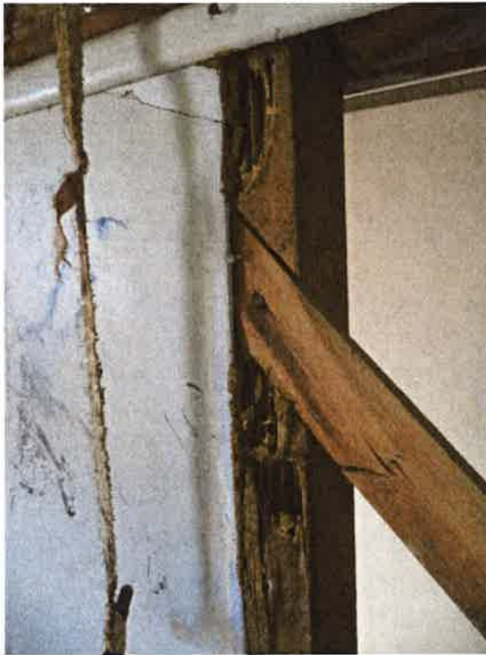
Figure 30: Detailed views of severely termite affected timbers
