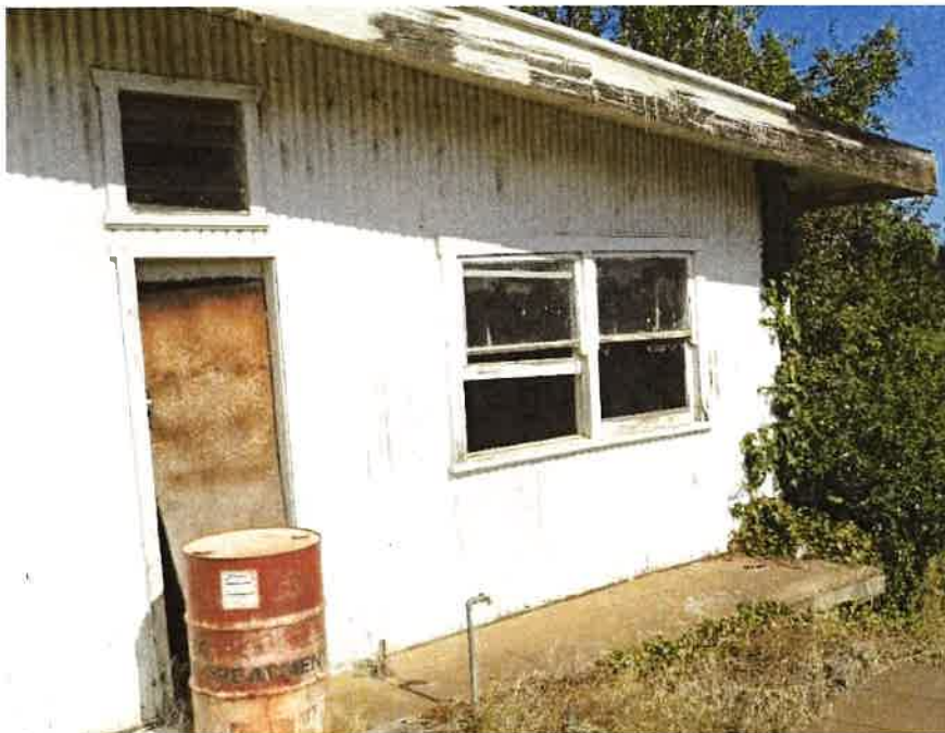
Figure 26: Detailed view of damaged cladding and timber, broken windows and door is boarded up
