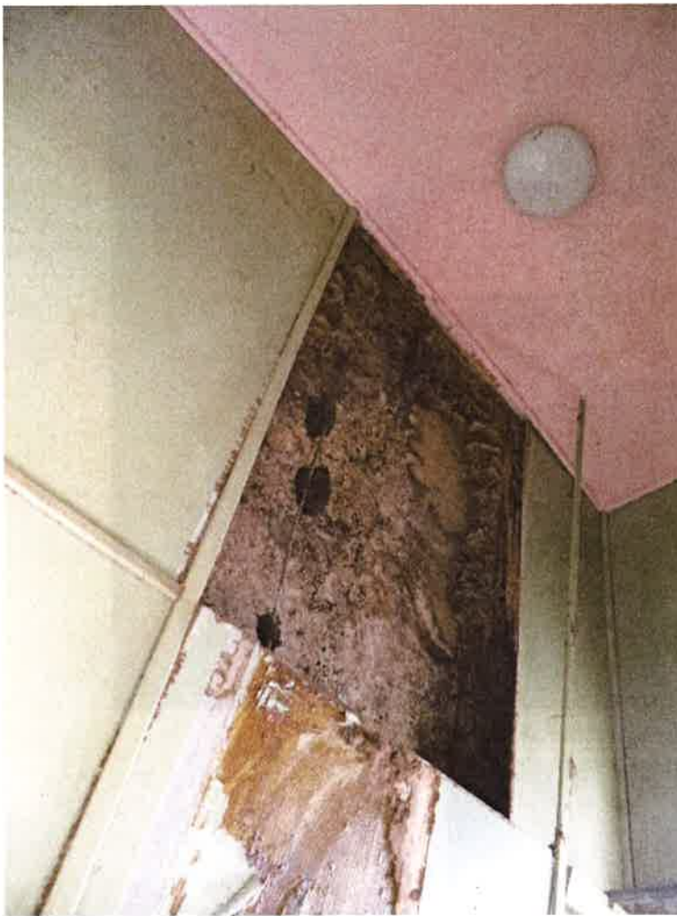
Figure 34: Fallen cladding exposing termite nests and damage to structural materials
