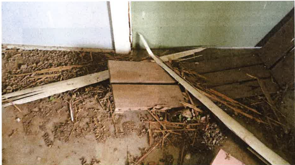
Figure 31: Detailed view fallen timbers and termite detritus
