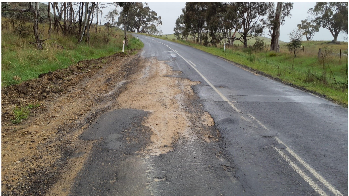
Photo of Icely Road, damage from spring to sealed road
