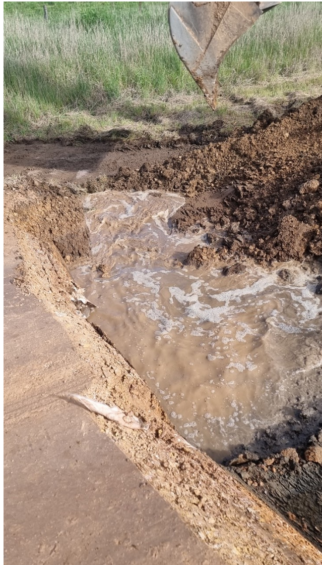
Photo of water from spring flowing out of sealed road while repairs are underway
